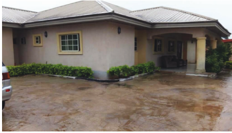
FIGURE 1: House side view.
