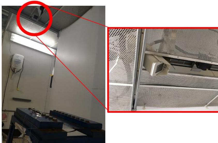
Figure 7.1:4 – Camera installed over flat plate setup
