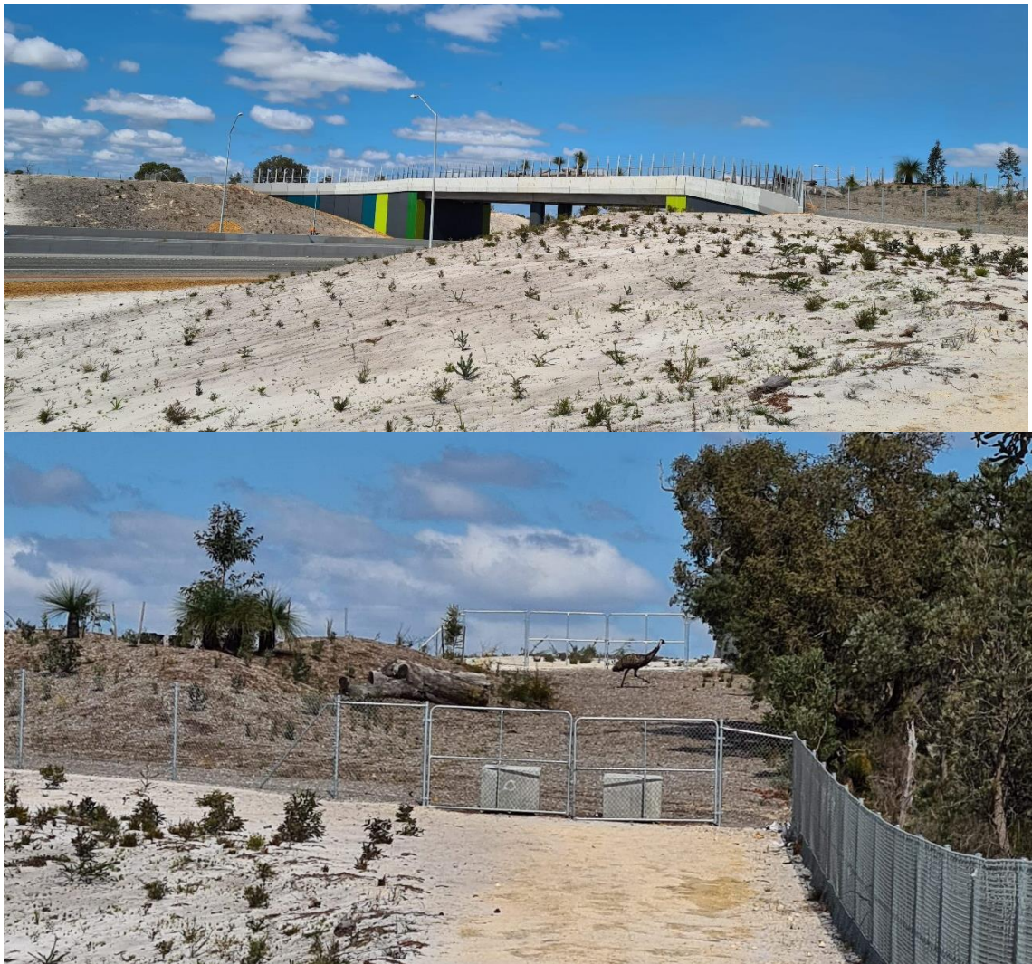
Figure 30. The fauna bridge over Tonkin highway links two IUCN class a1 nature reserves and is large enough to allow larger species movement (top) and an emu demonstrating how to use the fauna bridge (bottom). Image supplied by author.
