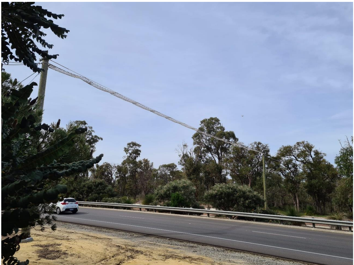
Figure 29. The possum bridge over Beeliar Drive connecting the Beeliar wetlands, over which possum movement would otherwise be hindered by this road barrier. Image supplied by author.
