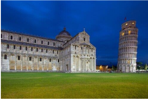
Leaning Tower of Pisa
