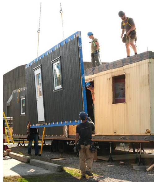
Figure 2. Pilot Retrofit at Bells Corners.
