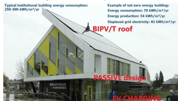
Figure 1. Varennes Library – Canada's first institutional NZEB with a building integrated photovoltaic/thermal system, passive solar design, EV charging, a geothermal heat pump system and radiant slabs.
