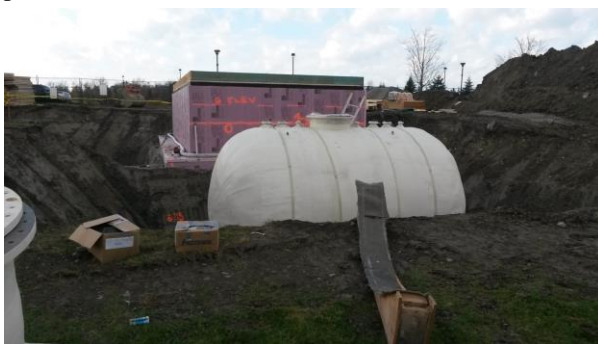
Figure 5. Seasonal store in ground next to basement of unfinished house.
