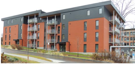
Figure 1. Picture of the case study building.
