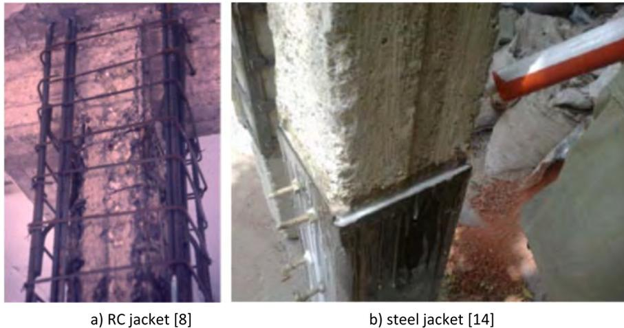
Fig. 3. RC columns repair using RC and steel jackets. a) RC jacket [8] b) steel jacket [14].
