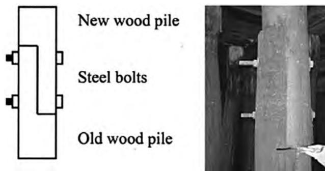
Fig. 2. Splicing of timber piles [21].
