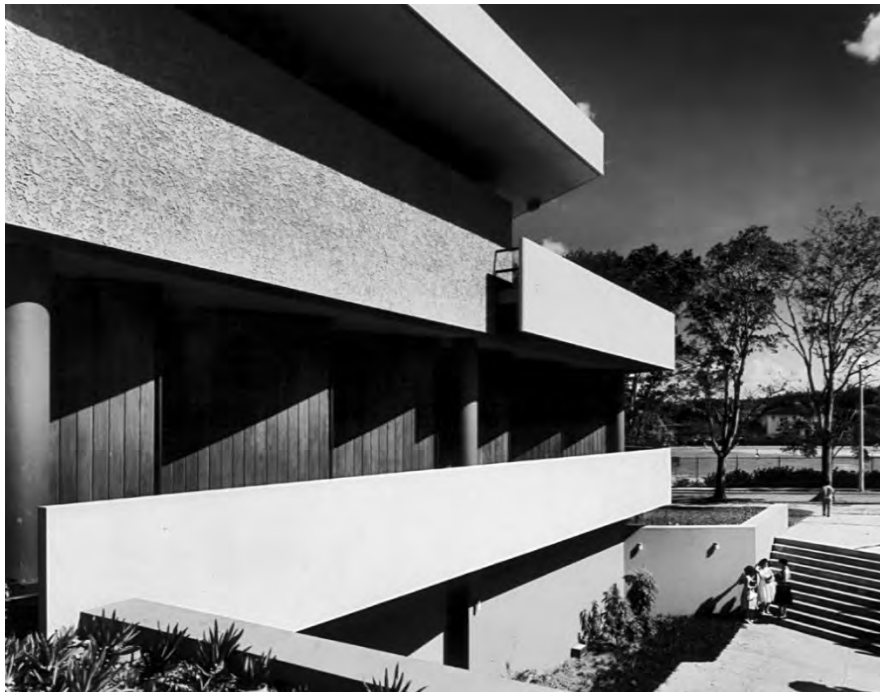
Figs. 3.7 & 3.8 – The Colegio San Ignacio de Loyola (1952) & Centro de Estudiantes/Student Hall at the University of Puerto Rico, Río Piedras Campus (1958) both features the “Stippled Cement Plaster Finish.” Source: Henry Klumb Collection, AACUPR.
