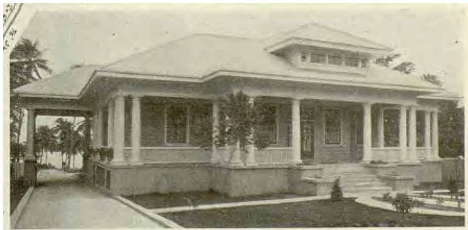
Fig. 1.5 & 1.6 – Wealthy American investors also landed in Puerto Rico in the early 1900s, preferring the use of reinforced concrete as the 'modern and material of progress.' It was also in Condado and Miramar where residences were built in the 'cottage' or 'bungalow' style using reinforced concrete techniques and concrete blocks such as 'Compo Stone.' The house of prominent Architect Antonin Nechodoma who praised the use of reinforced concrete in the early twentieth century (top photo) & House of Mr. J.B. Diaz, today known as Casa Benítez in Miramar (bottom photo). Source: Building Age , August 1918, Vol. 40, No. 8, p. 396.
