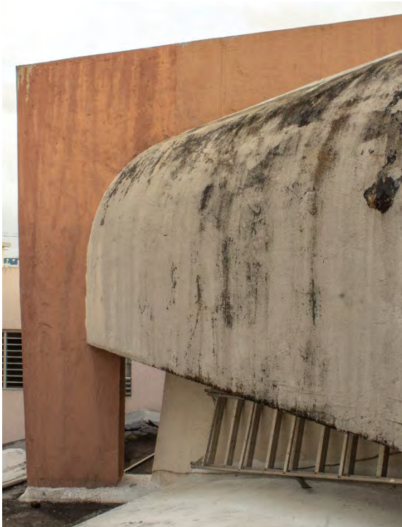
Figs. A2.71 & A2.72 – Discoloration, fouling and paint peeling conditions on Column A (left). Small detachment/debonding area behind Column A (right). Photos by Author, 2020.
