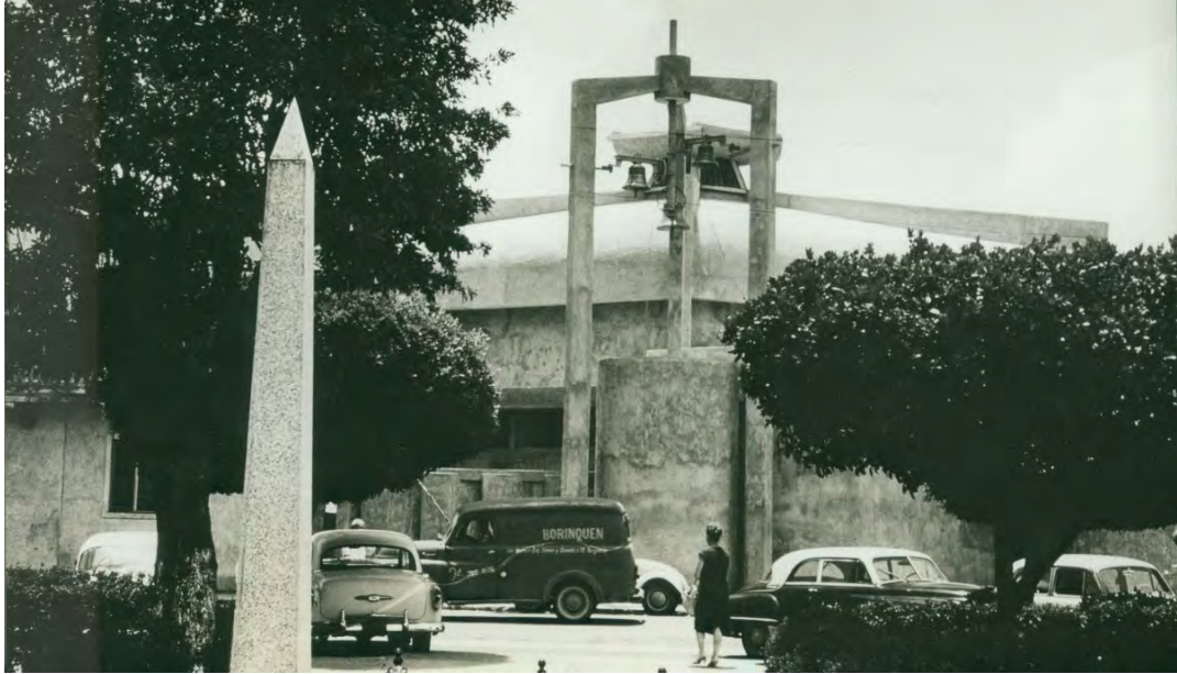
Fig. 4.19 – Del Carmen Church before inauguration in 1963. The differences in stuccoed surfaces can be seen also in the bell tower. Source: Henry Klumb Collection, AACUPR.
