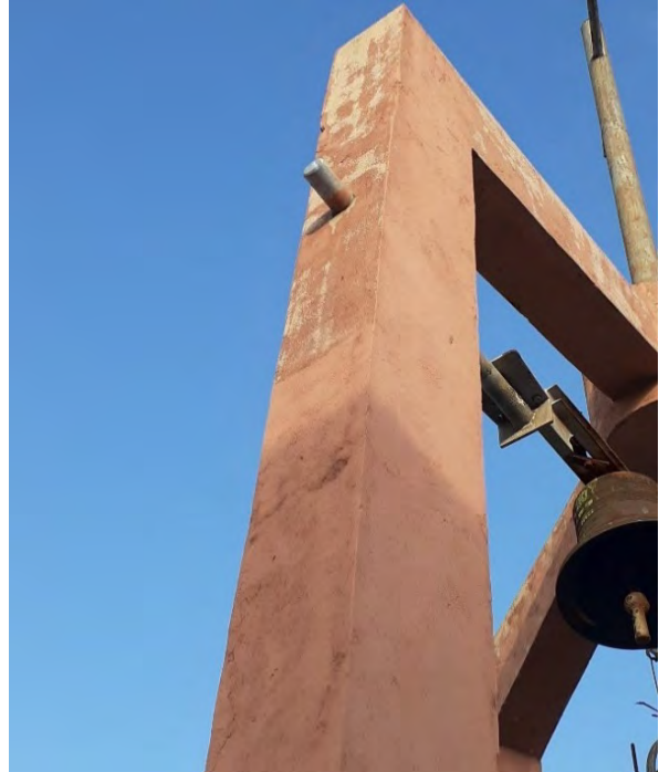
Figs. A2.49 & A2.50 – Improper repairs, paint peeling, discoloration, humidity and possible alkali-aggregate reaction (AAR) issue (as defined by Poole & Sims, 2016) on Elevation 11C of the belfry. Photos by Author, 2020.
