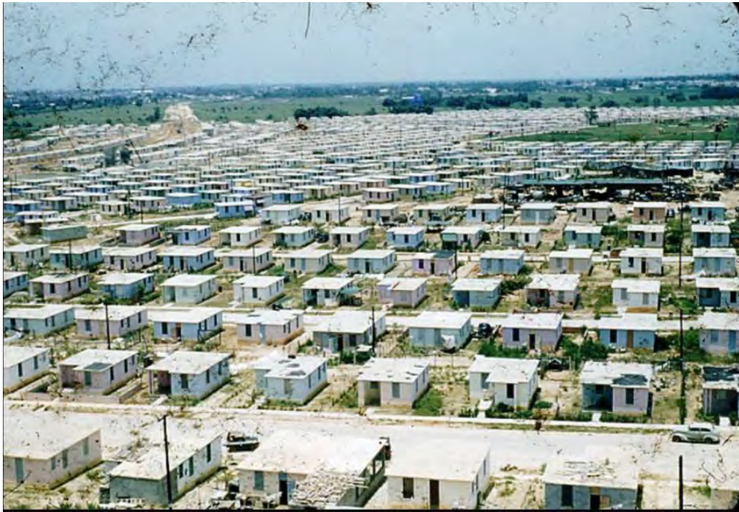
Fig. 1.13 – Bay View in Cataño and Puerto Nuevo in San Juan became pioneering private suburban developments with the construction of hundreds of plain and unornamented housing units with flat roofs and horizontal elements in their design. Using reinforced concrete (quick, portable, easy to use, and inexpensive construction system, and also as the 'clean and sanitary' building material), these residential typologies paved the way for future modern residential units in Puerto Rico. Photo of the Urbanización Puerto Nuevo seen from the San Patricio area c.1949. Source: Héctor Ruiz, "Urbanización Puerto Nuevo-1949", Redescubriendo a Puerto Rico Blog, March 13th, 2013, https://redescubriendopuertorico.blogspot.com/2013/03/urbanizacion-puerto-nuevo-1949.html
