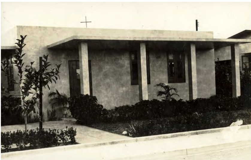
Figs. 3.26, 3.27 & 3.28. Suburban houses developed by the Puerto Rico Reconstruction Administration (PRRA) at the Urb. Eleanor Roosevelt in Hato Rey, San Juan (1937) with a smooth portland cement stucco finish. Source: Colección Digital Biblioteca Escuela de Arquitectura – Universidad de Puerto Rico, Recinto de Río Piedras (UPRRP).
