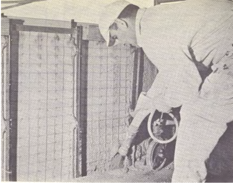
Fig. 3.15 & 3.16 – Dry-mix application of Shotcrete in the 1960s. Fig 6 shows the use of a hand hopper machines was also common in the era, suitable for sprayed finish coats. Source: Manual of Lathing and Plastering by John R. Diehl (1960), p. 176 & 91.
