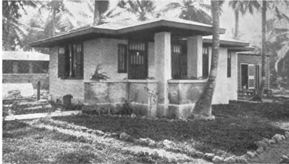
The composition of the concrete gives a pleasing texture to the finished surface.
