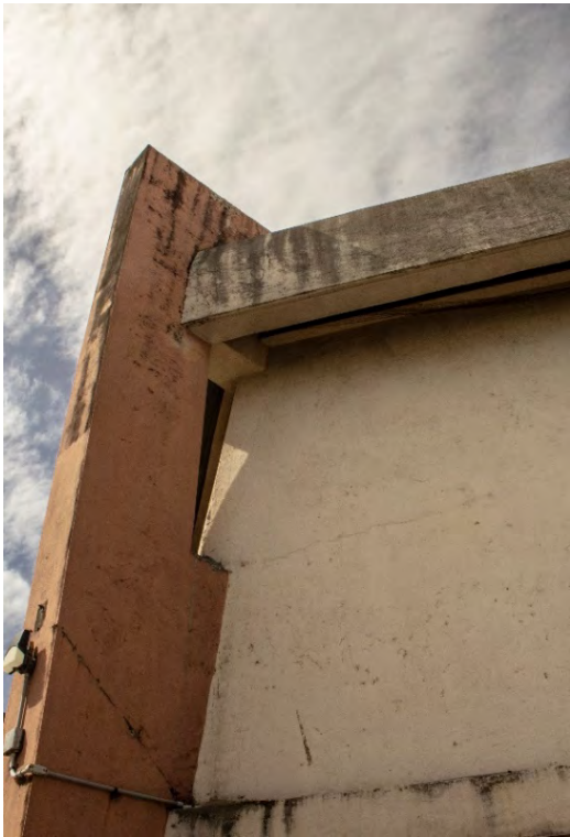
Fig. A2.85 & A2.86 – Fouling, mold growth and scaling of the surfaces along Column D (left photo). The largest detaching/debonding area on a structural column in the Church is seen on the back of Column D Photos by Author, 2020.
