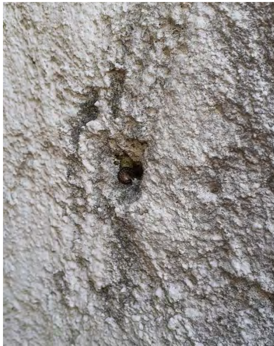
Figs. A2.10, A2.11 & A2.12 - Water ponding due to the new drainage along poor water management issues have increased the chance of development of micro and macro biogrowth on Side B of Elevation 3. These include mold growth, leafy plants and insects living on scaled stucco. Photos by Author, 2020.
