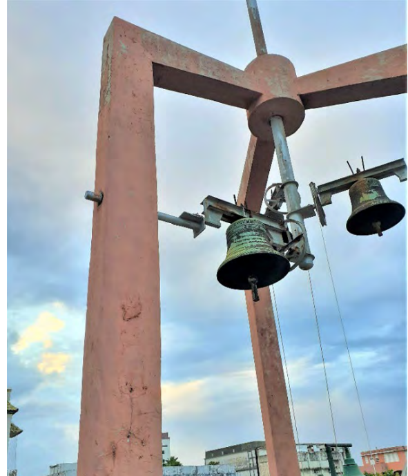
Figs. A2.47 & A2.48 – Diagonal cracking, discoloration, scaling and paint peeling issues on reinforced concrete masonry belfry. Photos by Author, 2020.
