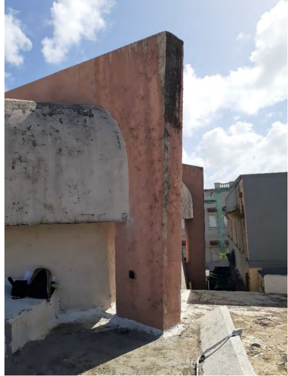
Fig. A2.75 & A2.76 – Detachment/debonding areas on the back of Column B. Other conditions include scaling, discoloration, fouling, mold growth and paint peeling. A corroded electrical metallic socket can be seen on the lower part of the column. Photos by Author, 2020.
