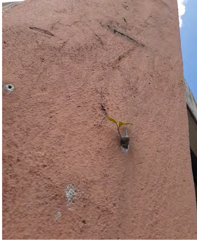
Fig. A2.90 – Small leafy plants growing along the stuccoed surfaces of Column E. Photos by Author, 2020.
