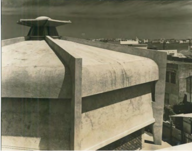
Fig. 1.29 – The Del Carmen Church in Cataño (1962). Source: AACUPR – Klumb Collection.
