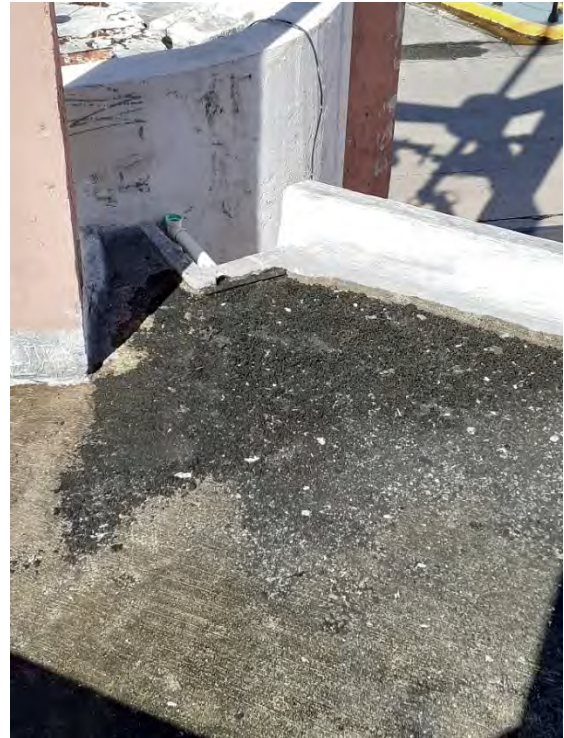
Figs. A2.39 & A2.40 – A broken drainage from building on the west side of the church creates a massive water ponding issue on the roof slab. The two original 'Type B' drains are not working (left photo). New installed drainage which leads to water ponding, increasing moisture and bio-growth issues on Elevation 3. This new drainage is the only one properly functioning on the roof (right photo). Photos by Author, 2020.
