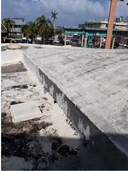
Fig. 4.15 & 4.16 – Sealing roof paint & waterproof coating conditions at the Del Carmen Church. Photos by Author, 2020.
