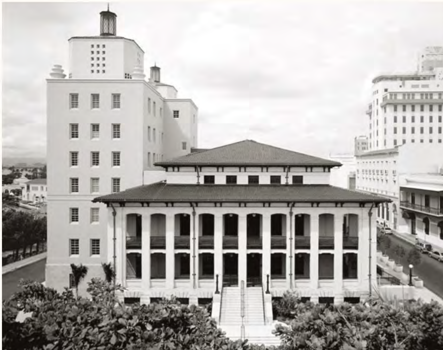
Fig. 1.2– The Federal Building and U.S. Courthouse in Old San Juan, built-in 1914, was the first and most expensive federal building constructed in Puerto Rico during this period. As the southern edge of an old ashlar, rubble and brick masonry city, the building was a symbol of the new colonial order which used the reinforced concrete system. Source: H. Santiago and F. J. Del Campo, “US Post Office and Courthouse/Old San Juan Federal Building” National Register of Historic Places Inventory/Nomination Form , March 28th, 1988.
