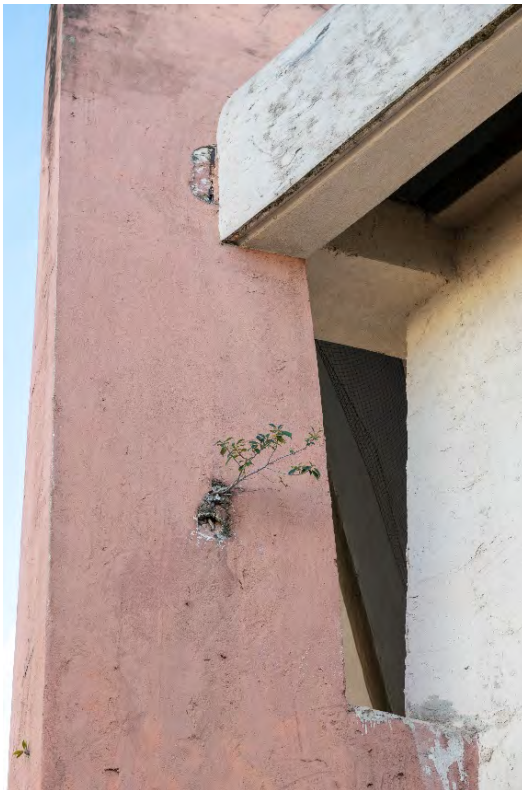
Figs. A2.91 & A2.92 – Scaling and leafy plants growing on the stucco surfaces of Column E. Lamps have been installed on Columns D, E and F, attaching them to the stuccoed surfaces. Photos by Author, 2020.
