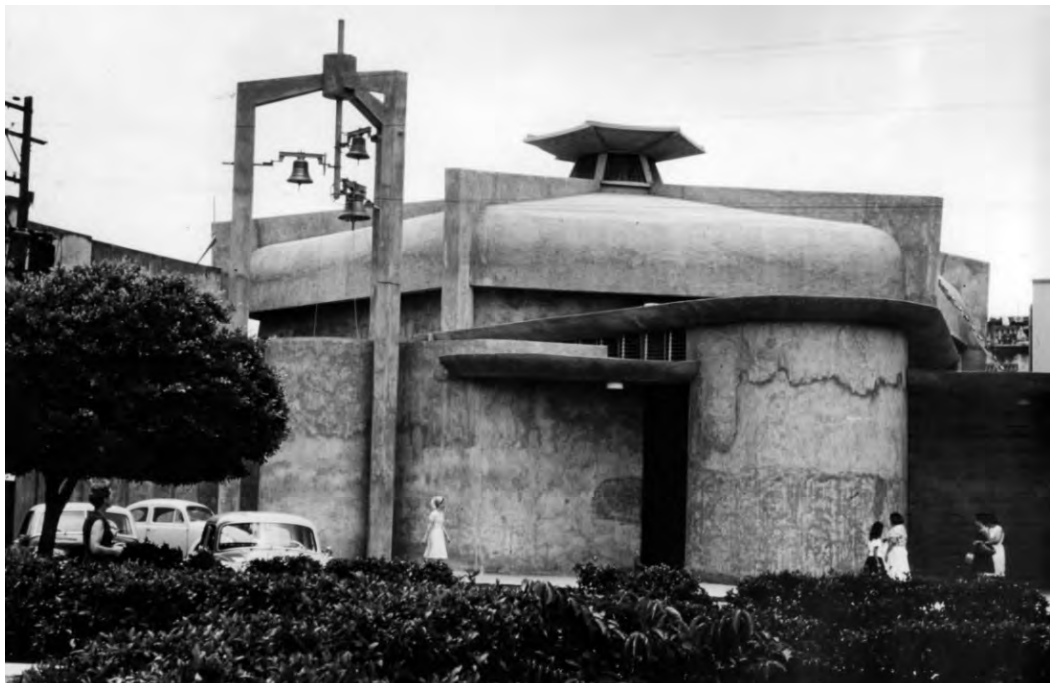
Fig. 4.18 – Del Carmen Church before inauguration in 1963. The differences in the concrete masonry surfaces are evident vs. the dome finish. Source: Henry Klumb Collection, AACUPR.
