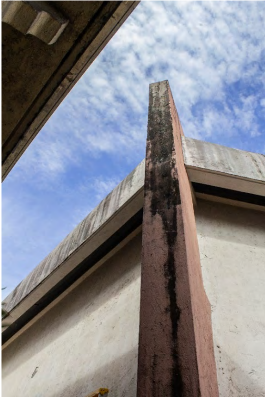
Fig. A2.81 & A2.82 – Surface fouling, mold growth and paint peeling on Column C (left photo). Small detaching/debonding areas on the base of Column C (right photo). Photos by Author, 2020.
