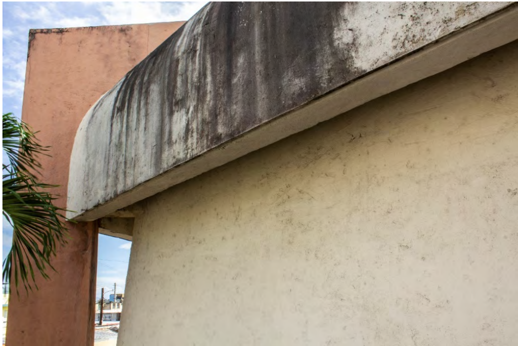
Fig. A2.95, A2.96 & A2.97 – A failing previous repair behind Column F (top left photo). Fouling, scaling and vertical/horizontal cracking issues on the top of Column F (top right and bottom photos). Photos by Author, 2020.
