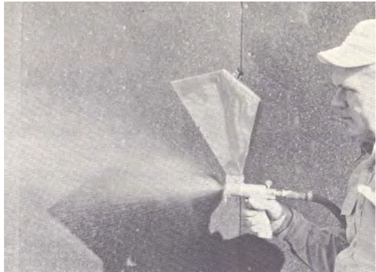
Fig. 3.15 & 3.16 – Dry-mix application of Shotcrete in the 1960s. Fig 6 shows the use of a hand hopper machines was also common in the era, suitable for sprayed finish coats. Source: Manual of Lathing and Plastering by John R. Diehl (1960), p. 176 & 91.
