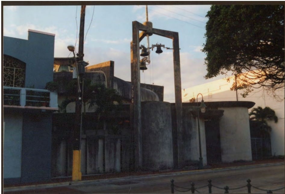
Fig. 4.23 & 4.24 – Del Carmen Church c.1999. Atmospheric soiling and bio-growth on the exposed surfaces before the painting campaigns of the 2000s. It is possible that a coat of paint was applied in the late 1990s to address surface disfigurement. Source: R. Otero
