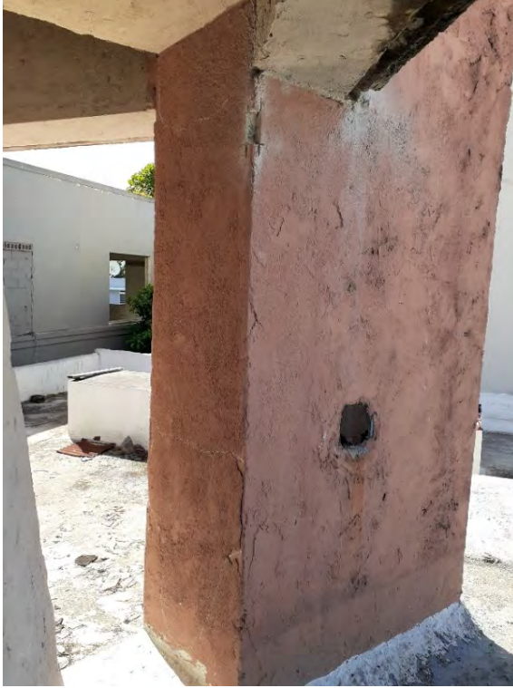
Fig. A2.75 & A2.76 – Detachment/debonding areas on the back of Column B. Other conditions include scaling, discoloration, fouling, mold growth and paint peeling. A corroded electrical metallic socket can be seen on the lower part of the column. Photos by Author, 2020.
