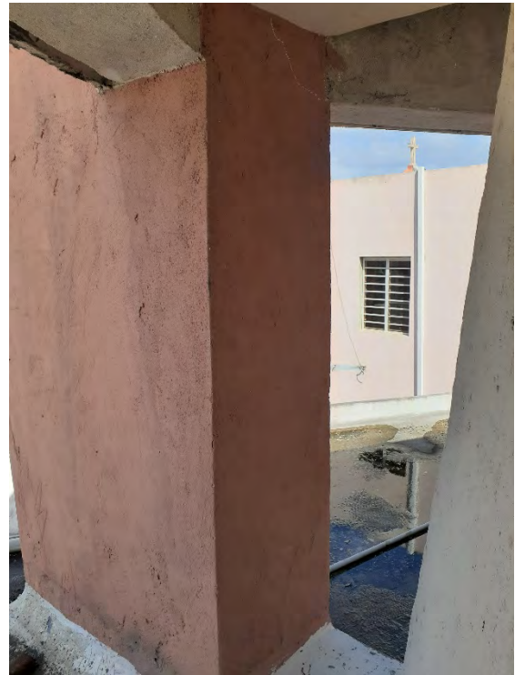
Figs. A2.71 & A2.72 – Discoloration, fouling and paint peeling conditions on Column A (left). Small detachment/debonding area behind Column A (right). Photos by Author, 2020.
