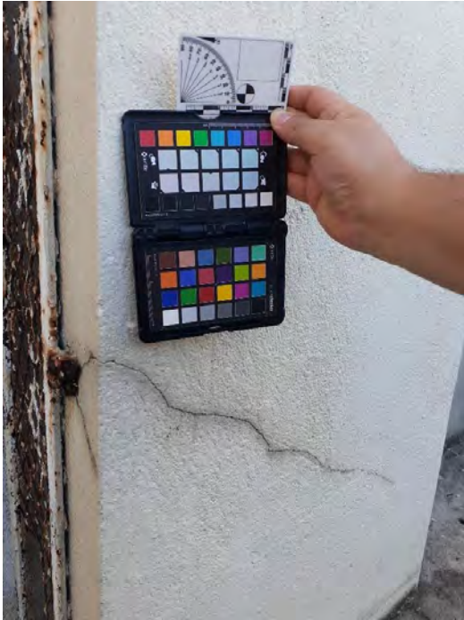
Fig. 4.8 & 4.9 – Condition issues on precast wall (north side) and the stuccoed cast-in-place wall on the southeast side of the church. Photos by Author, 2020.
