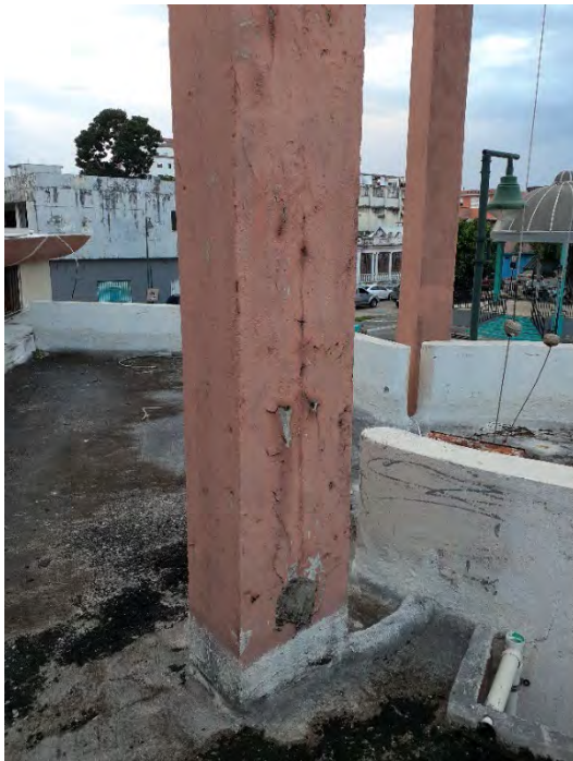
Figs. A2.49 & A2.50 – Improper repairs, paint peeling, discoloration, humidity and possible alkali-aggregate reaction (AAR) issue (as defined by Poole & Sims, 2016) on Elevation 11C of the belfry. Photos by Author, 2020.
