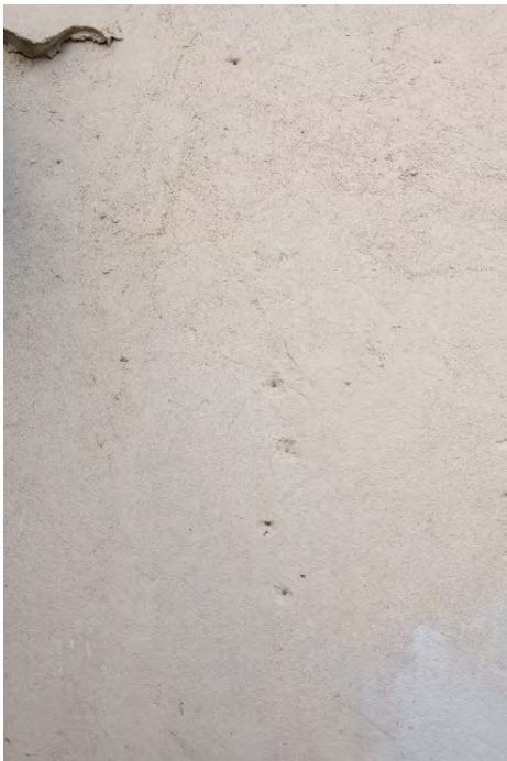
Fig. A2.30 & A2.31 – Scaling of stucco and corrosion staining over the surfaces of Elevation 7. Photos by Author, 2020
