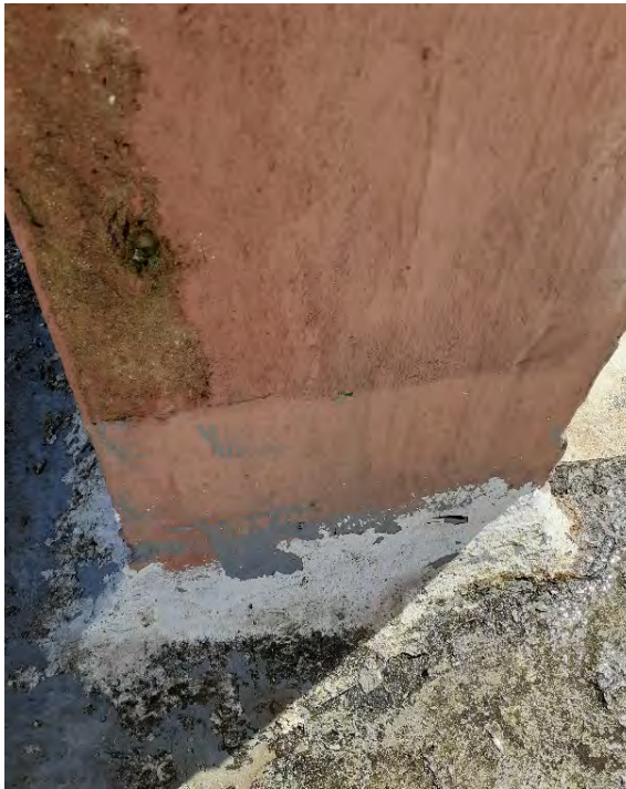
Fig. A2.77 & A2.78 – The roof sealing paint was applied to the base of both Column B and Column A. Also, the gray sealing coating was applied in the upper parts of the column (see the differences in layers). Photos by Author, 2020.
