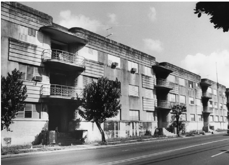
Figs. 3.29, 3.30 & 3.31 -The house of architect Antonin Nechodoma in Miraflores, Santurce (built c.1913) & El Falansterio Housing, designed by Architect Jorge Ramírez de Arellano for the Puerto Rico Reconstruction Administration (PRRA) in 1937. These two are examples of the experimentation with early 'fair-faced' exposed concrete in Puerto Rico between the 1900 and 1940. Source: AACUPR.
