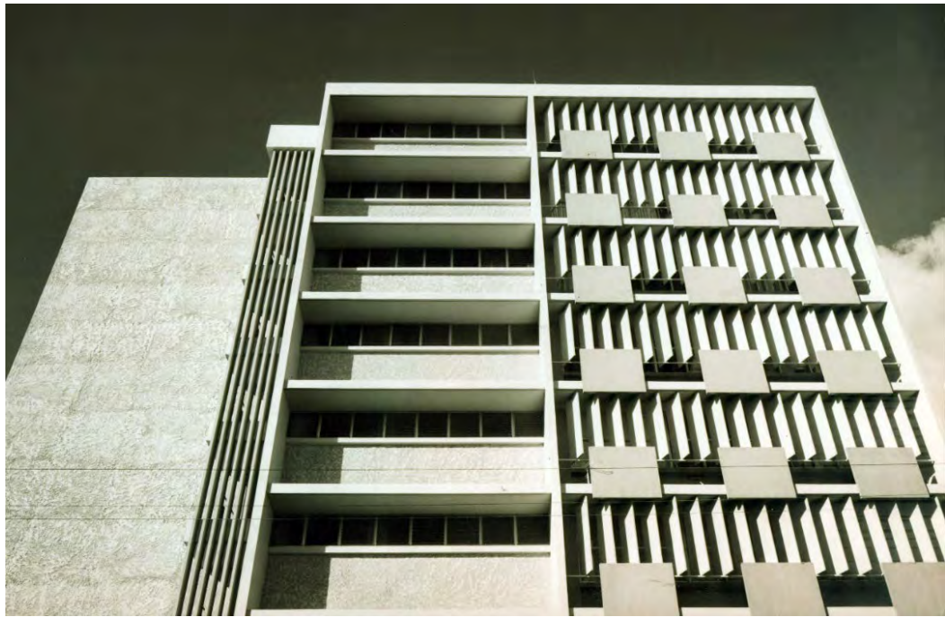
Fig. 3.5 – The San Martín Office Building & Condominium, Santurce (1957) featured the use of the “Rough Cement Plaster Finish” on the building’s exteriors. Source: Henry Klumb Collection - AACUPR
