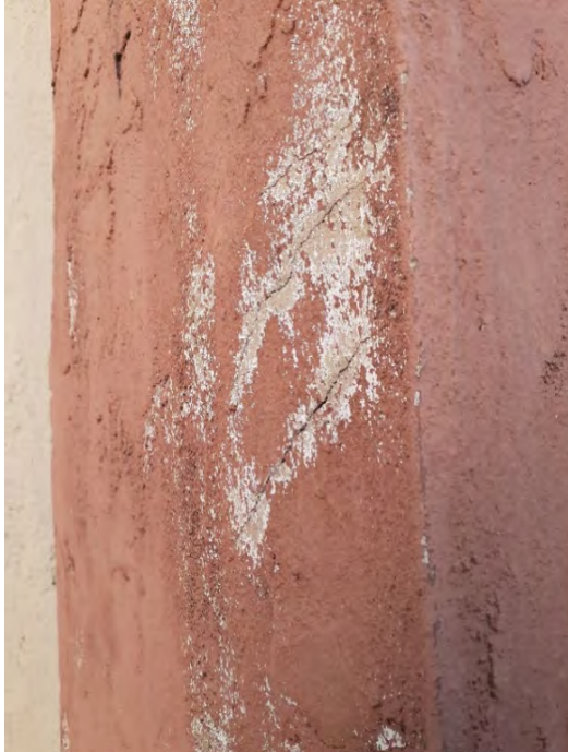
Figs. A2.47 & A2.48 – Diagonal cracking, discoloration, scaling and paint peeling issues on reinforced concrete masonry belfry. Photos by Author, 2020.
