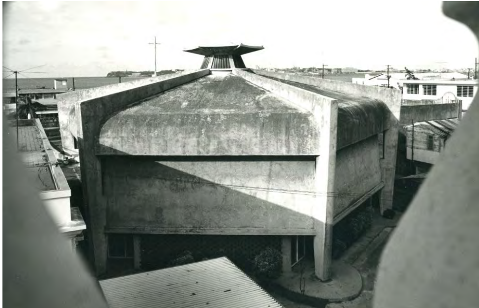
Fig. 4.22 – Del Carmen Church c.1965. Extensive surface fouling issues in the form of black bio-growth has been present in the dome since its early days. Source: Henry Klumb Collection, AACUPR.
