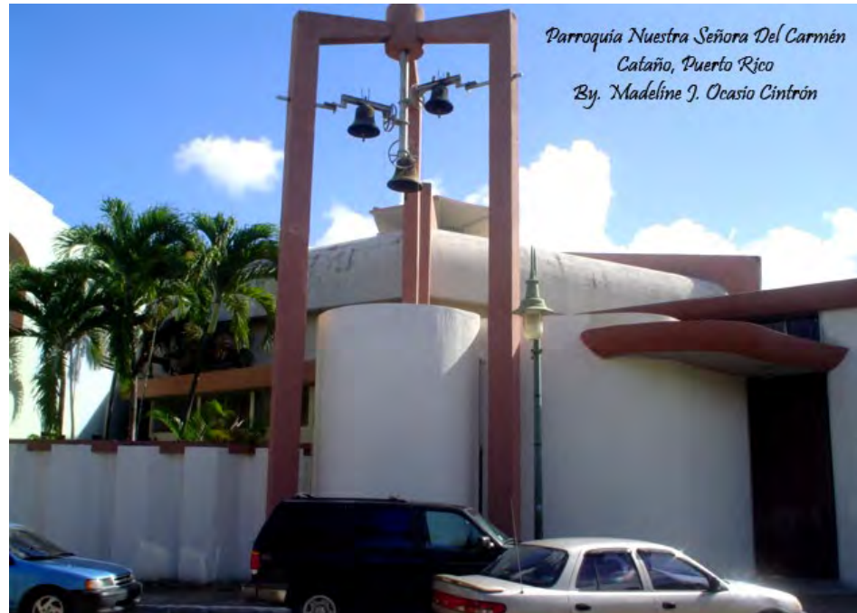
Fig. 4.25 – Del Carmen Church in 2006. All the concrete and stuccoed exterior surfaces after the second paint campaign. The first paint campaign was applied between the late 1990s and early 2000s. Source: Madeline Ocasio, Flickr.
