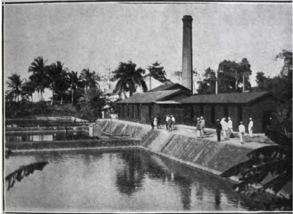
Fig. 1.1– Acueducto de Río Piedras/Río Piedras Aqueduct. At the time it had three enormous water tanks and an Industrial Mechanical Warehouse. The Aqueduct could filter more than 500,000 gallons of water daily at the time. Source: Puerto Rico Ilustrado, 1919.
