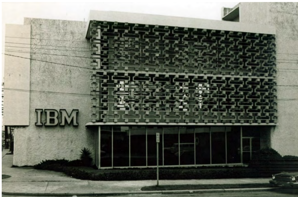
Figs. 3.2 & 3.3 – Elevation & Photo of the IBM Office Building for the San Juan Real Estate Corp., in Santurce (1958). Klumb featured the use of the “Rough Cement Plaster Finish” on the building’s exteriors. Source: Henry Klumb Collection - AACUPR
