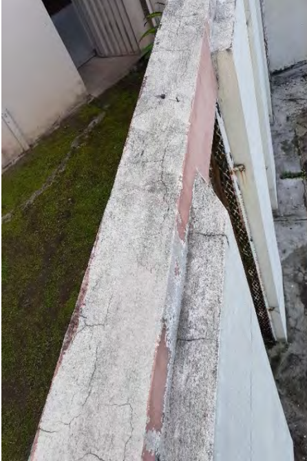
Fig. A2.26 & A2.27 – Cracking issues along the precast members of Elevation 6. Photos by Author, 2020.
