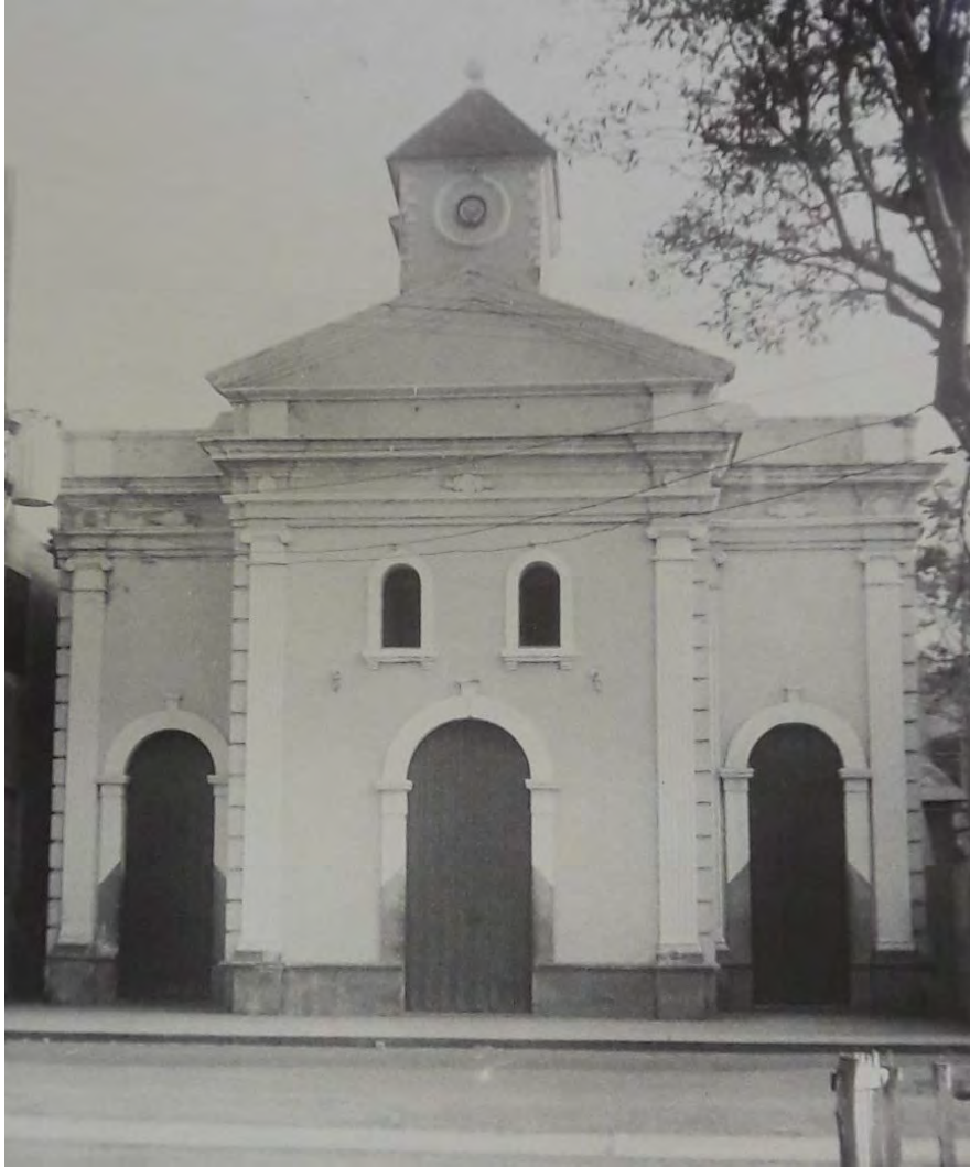
Fig. 2.15 – The old Del Carmen Church building from 1904-1905, c.1950. The belfry was seriously damaged by Hurricane Santa Clara in 1956 and was removed. Source: AACUPR – Henry Klumb Collection.
