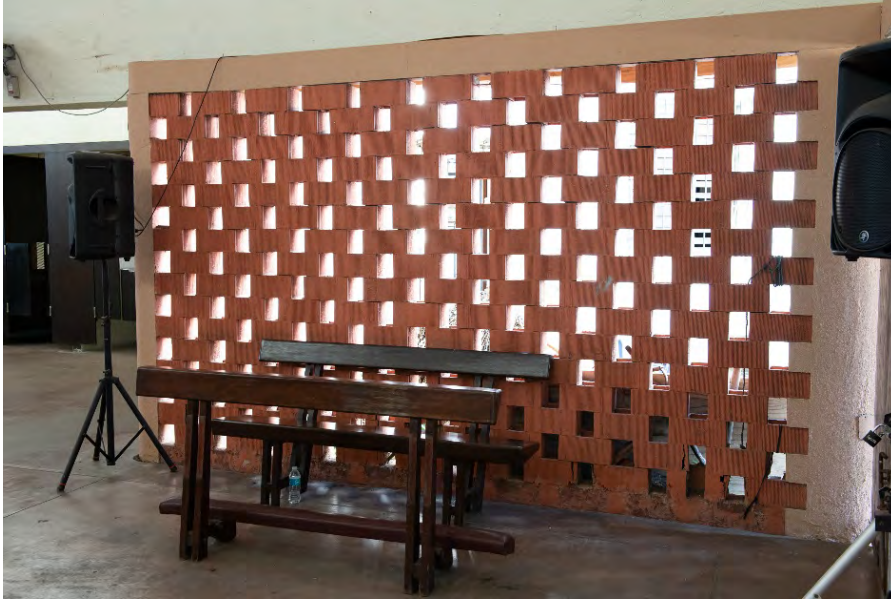
Figs. 2.38 & 2.39 – Terra cotta hollow block wall on the southeast side of the church, which allows a passive ventilation system and an interior-exterior connection (top photo). The entrance planter on the northwest side of the church (bottom photo). Photos by Javier Freytes, December 2019.
