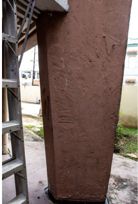
Fig. A2.81 & A2.82 – Surface fouling, mold growth and paint peeling on Column C (left photo). Small detaching/debonding areas on the base of Column C (right photo). Photos by Author, 2020.
