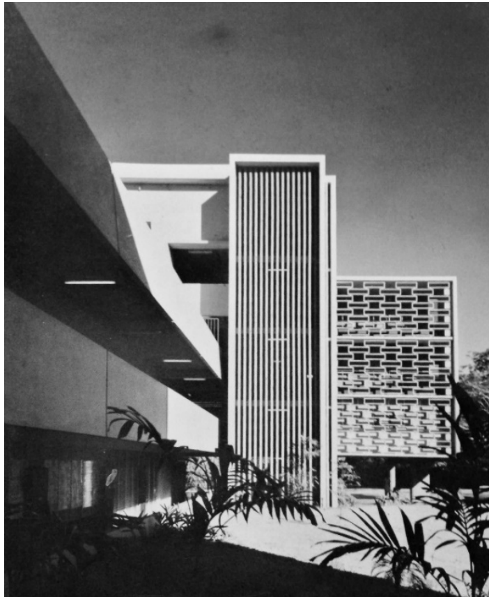
Fig. 2.3 – Social Science Faculty Building, UPR Río Piedras, San Juan, PR (1964). Source: AACUPR – Henry Klumb Collection.
