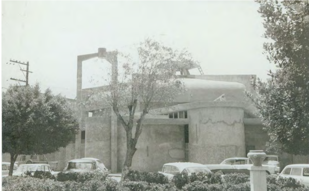
Fig. 4.17 – Del Carmen Church during construction in 1962. The variations on the stuccoed surfaces can be seen since the construction phase. Source: Henry Klumb Collection, AACUPR.
