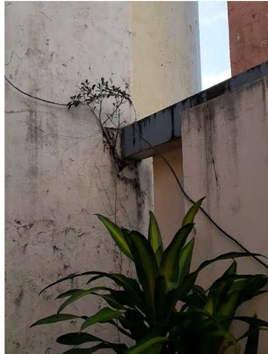
Figs. A2.10, A2.11 & A2.12 - Water ponding due to the new drainage along poor water management issues have increased the chance of development of micro and macro biogrowth on Side B of Elevation 3. These include mold growth, leafy plants and insects living on scaled stucco. Photos by Author, 2020.
