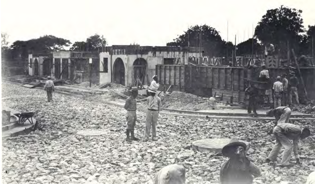
Fig. 1.8 – In the development of El Falansterio , the first Public Housing complex, and the Eleanor Roosevelt and Morel Campos suburban developments, the PRRA promoted hundreds of structures using reinforced concrete with simple design and flat roofs, which led to the quick production of these buildings. Photo of the Urbanización Morell Campos in Ponce under construction. Source: Biblioteca Digital Puertorriqueña, University of Puerto Rico-PRRA Collection.
