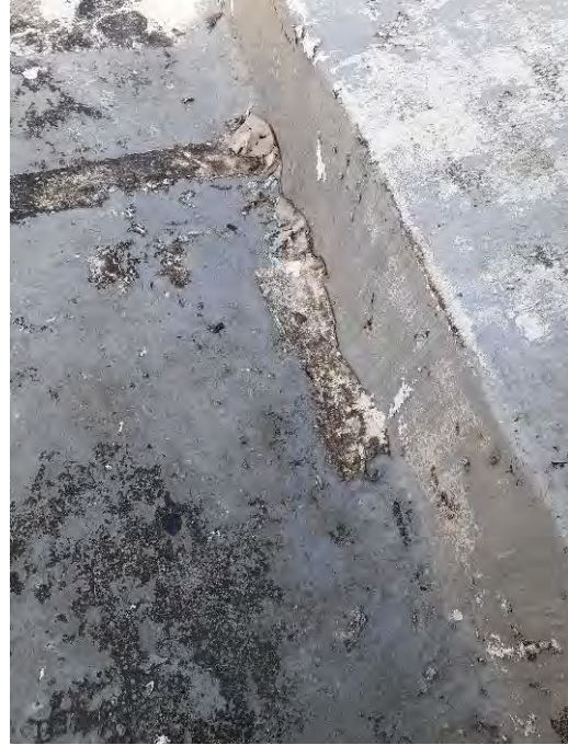
Fig. 4.15 & 4.16 – Sealing roof paint & waterproof coating conditions at the Del Carmen Church. Photos by Author, 2020.
