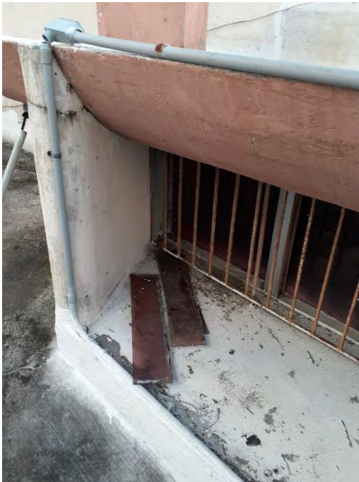
Figs. A2.42 & A2.43 - The original glass louvers can be found at the roof (left photo). Cracking, an improper repair and discoloration of the eaves in Elevation 10A (right photo). Photos by Author, 2020.
