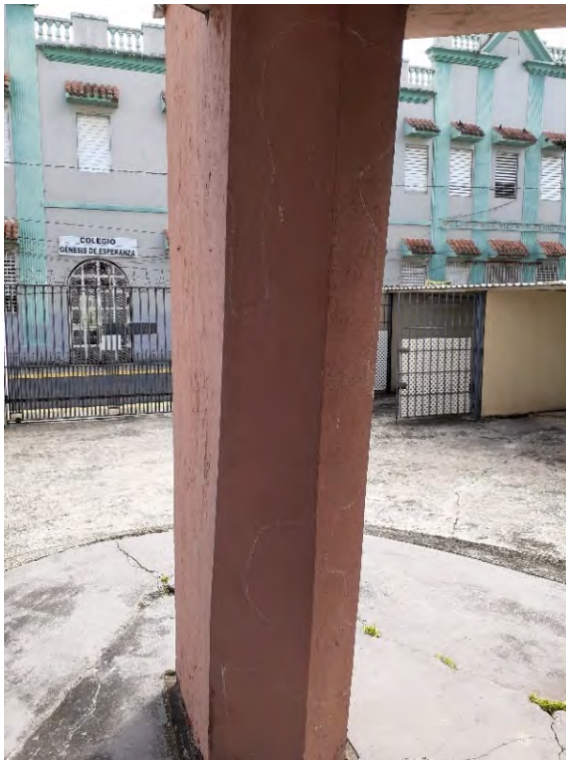
Fig. A2.85 & A2.86 – Fouling, mold growth and scaling of the surfaces along Column D (left photo). The largest detaching/debonding area on a structural column in the Church is seen on the back of Column D Photos by Author, 2020.
