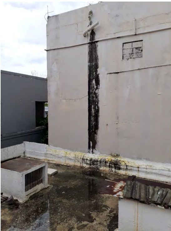
Figs. A2.39 & A2.40 – A broken drainage from building on the west side of the church creates a massive water ponding issue on the roof slab. The two original 'Type B' drains are not working (left photo). New installed drainage which leads to water ponding, increasing moisture and bio-growth issues on Elevation 3. This new drainage is the only one properly functioning on the roof (right photo). Photos by Author, 2020.
