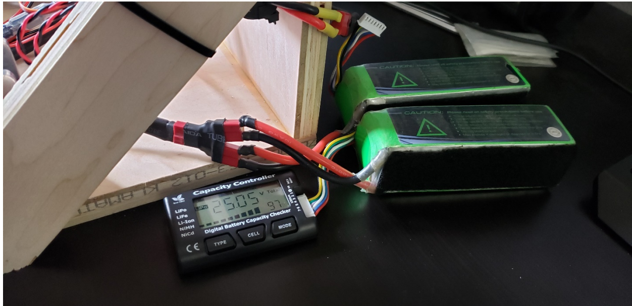
Figure 6.32 Main Battery Packs and Battery Monitoring
