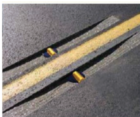
Figure 5.5 Installation of Banana Cut Marker (Dynatech, 2018).
