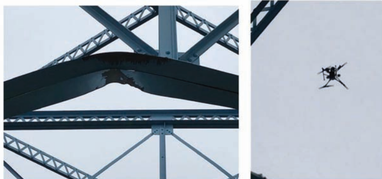
(a) UAS provides excellent vantage point to document bridge damage after bridge hit (Fitzgerald, 2020).
