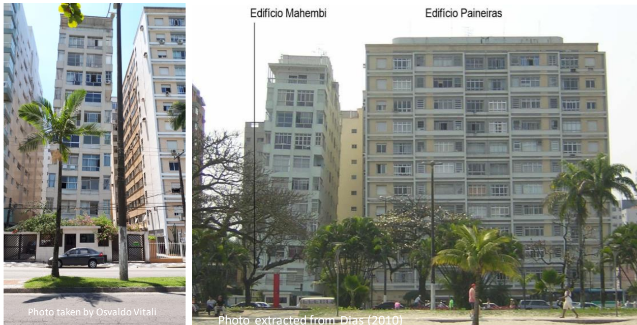
Figure 2. Photos of leaning buildings in Santos (on the left Mahembi building; on the right both Mahembi and Paineiras buildings).
