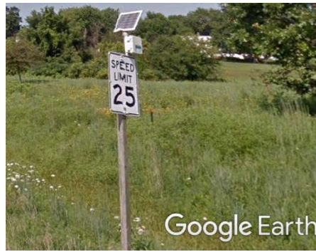
Speed limit with radar-activated LED lights (Hallmark et al., 2013).
