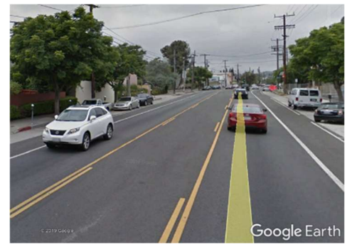
Road diet—reduce lanes from 4 to 3 (Corkle et al., 2001; FHWA, 2014; Knapp & Giese, 2001).
