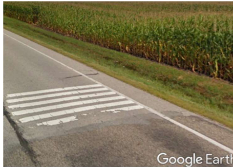
Rumble strips at high-speed intersections (FHWA, 2014; Ray et al., 2008).
