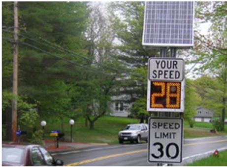
Speed feedback sign (Hallmark et al., 2013, 2007; Knapp & Giese, 2001) (Photo-Bagdade et al., 2012).
