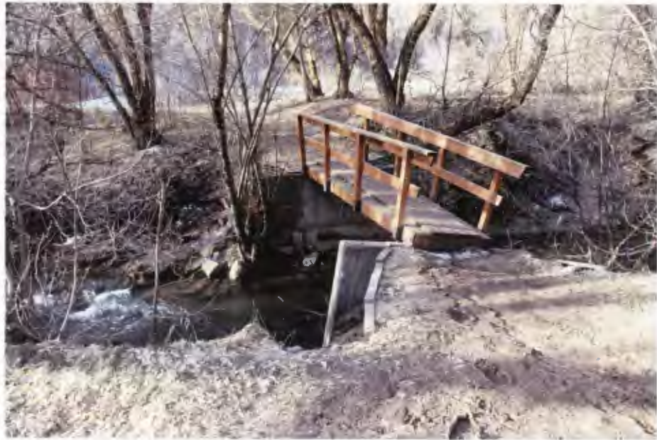
Figure 25. View of current bridge.
