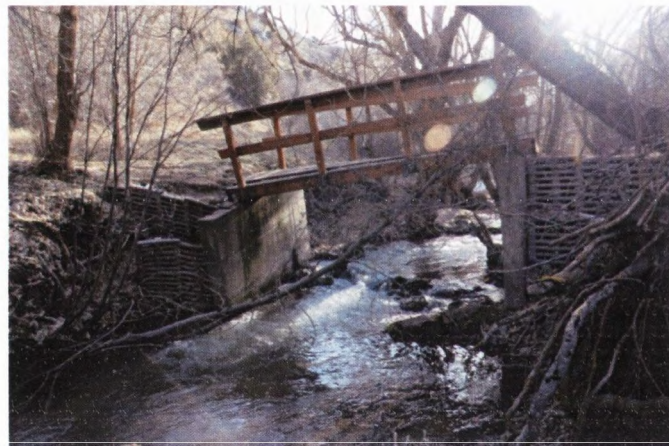
Figure 1. The condition of the existing bridge.
