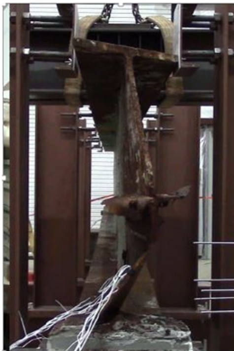
Figure 4.27: Residual Deformation of Corroded Web
