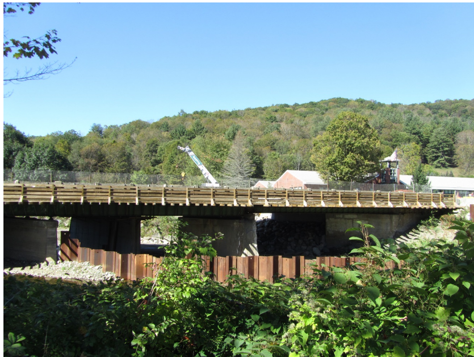
Figure 2.1: Bridge ID C18028-0KQ-DOT-NBI, Colrain, Massachusetts; approach span pictured on the right.
