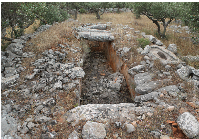
Figure 16. The large cistern in Koulouvades, looking west.
