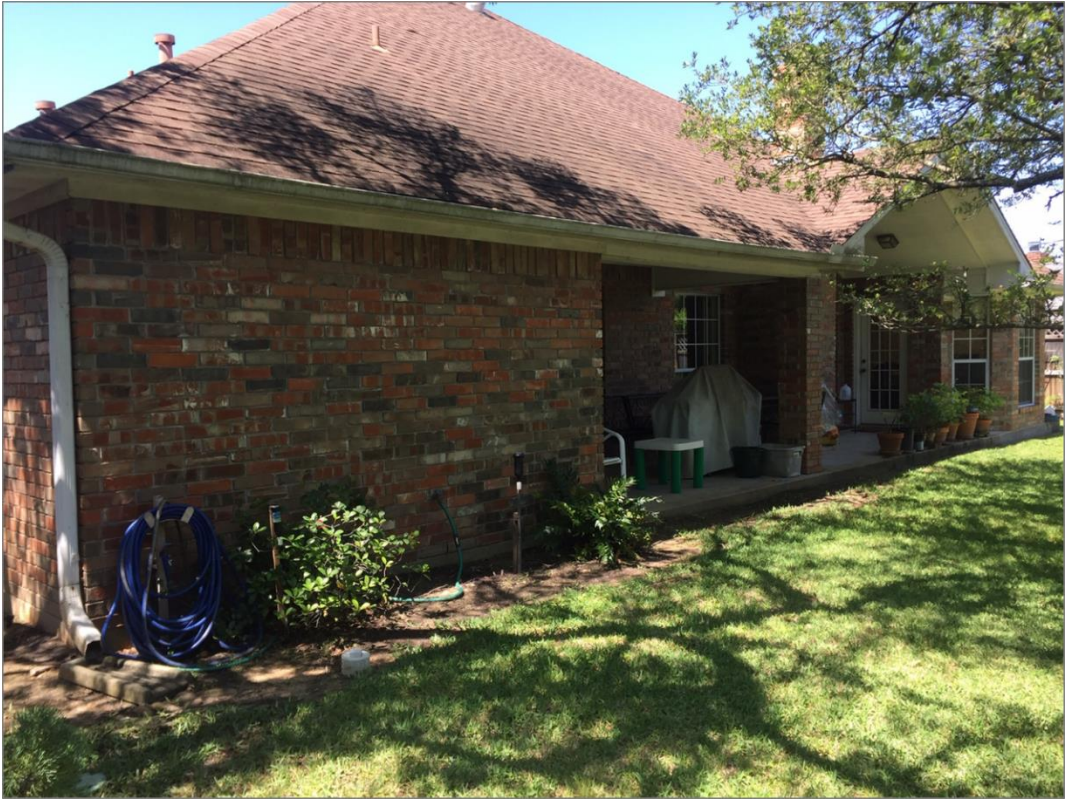
Figure 4.4: Back View (Northwest) of the Case-study House
