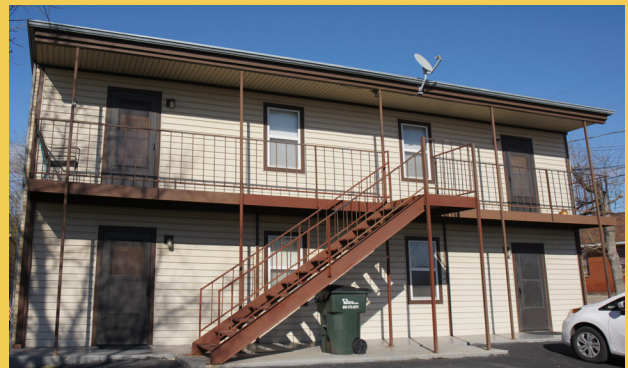
Figure 4.10 Apartments, Nolanville, TX Source: Google Maps, 2020
