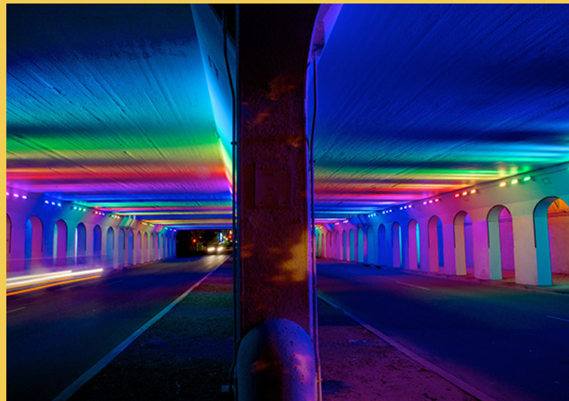
Figure 7.37 Underpass lighting by artist Bill FitzGibbons in Birmingham, AL Source: https://www.thisiscolossal.com/2013/08/bill-fitzgibbons-lightrails/
