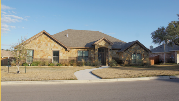
Figure 4.5 SF home, newer build, Nolanville, TX Photo by David Watson
