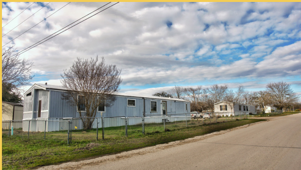
Figure 4.11 Manufactured home, Nolanville, TX Photo by David Watson
