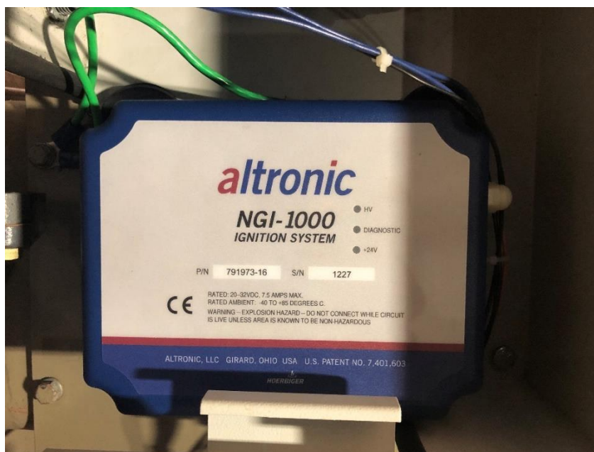
Figure 9: NGI-1000 ignition system mounted to Ajax E-565
