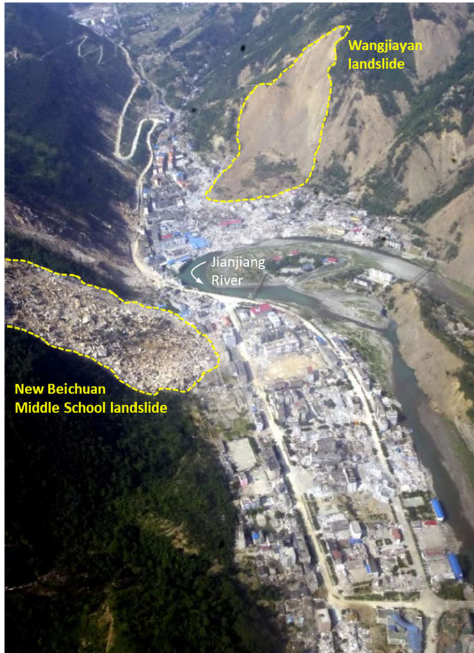
Figure 6.4 – Post-earthquake aerial image showing the ruins of the old Beichuan town (S-facing) (image: May 27, 2008; credit: Xinhua News Agency).
