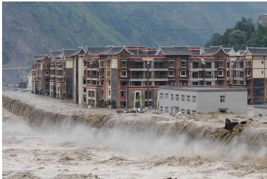
Figure 6.9 – Urban flooding in the reconstructed Yingxiu town during debris flow events on August 12-14, 2010 (image: August 15, 2010; credit: SKLGP).
