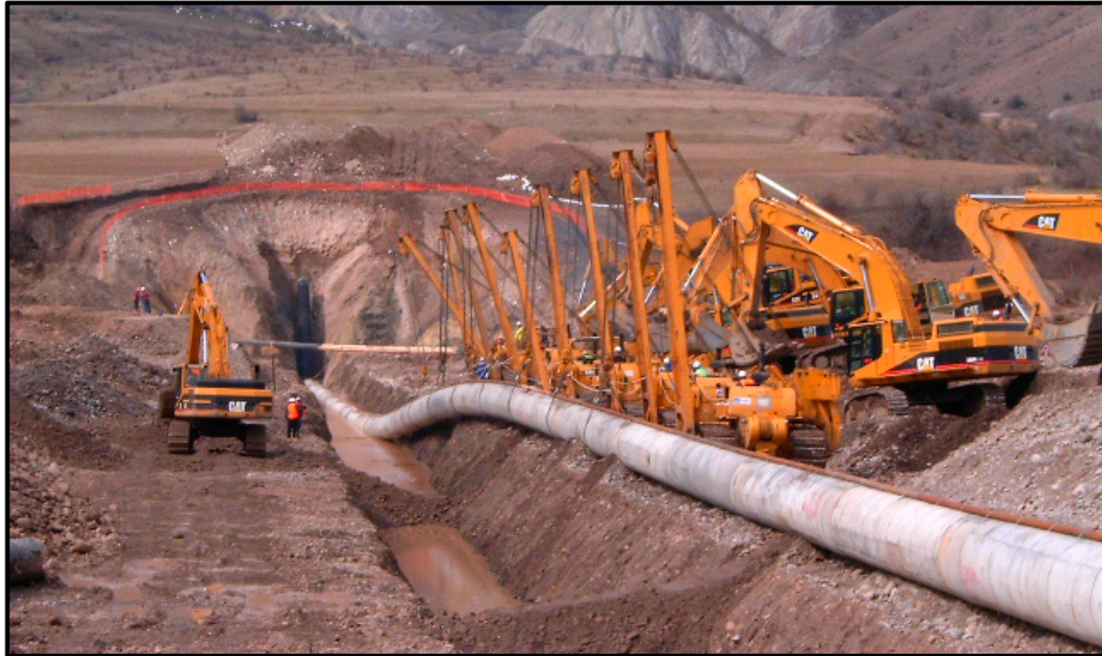
Figure 1.14 – Pipeline Lower and Lay (Georgia)
