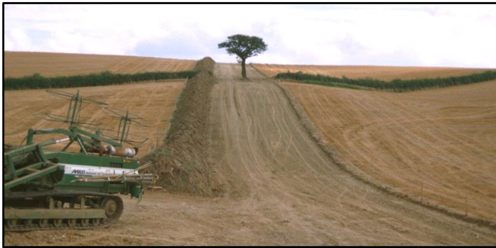
Figure 1.8 – Right of Way Preparation (UK)
