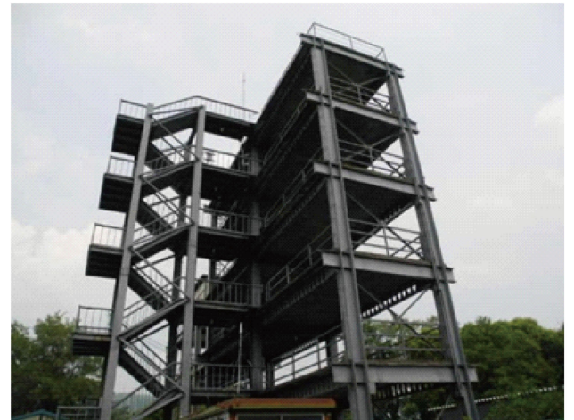
FIGURE 2 | Five-story steel building.
