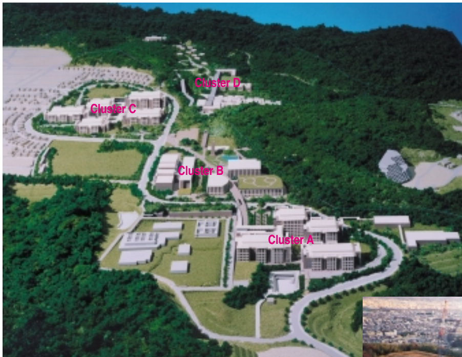
The scale model of the Katsura Campus. The campus consists of four clusters. The clearing of land has been kept to a minimum in the area of the site adjoining a bamboo grove in order to preserve a sense of harmony with the surroundings. The campus is aiming for certification to ISO 14001.
