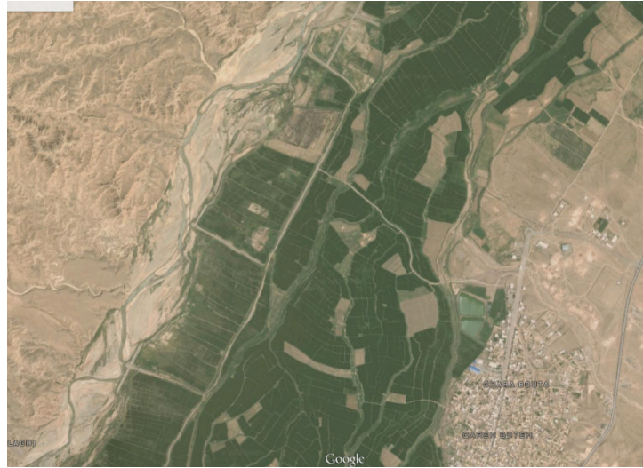
Figure 1-5. Spur dikes for protecting banks in Zanjanrood river, Iran (Image Courtesy of Google)
