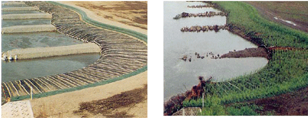
Figure 1-6. Spur dikes for landscape improvement and protecting banks in Tokachi river, Japan (Installation -left- and immediately after flood -right-) (Hong Koo 2007)
