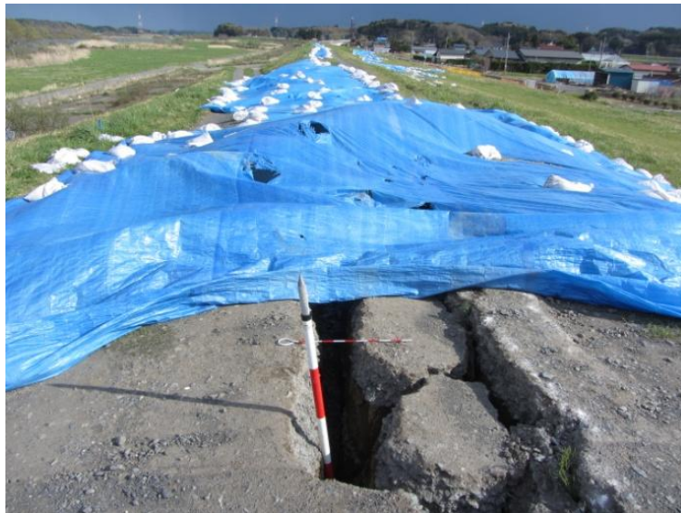
Figure 1.5. Naruse River right bank, Fukunuma (Oka et al., 2012)
