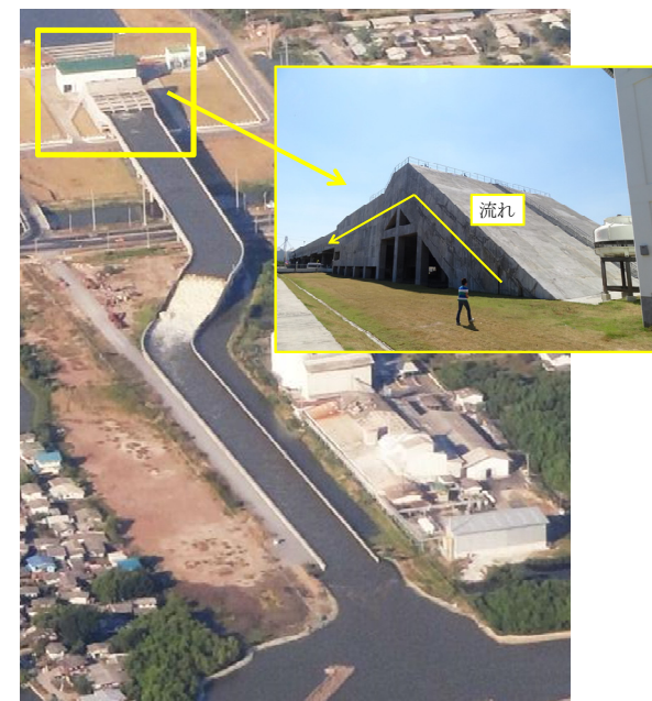
Fig. 3 Elevated canals near coastal area
