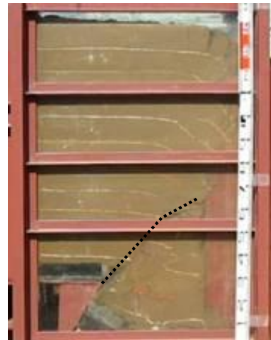
Photo 2 Fault part side
