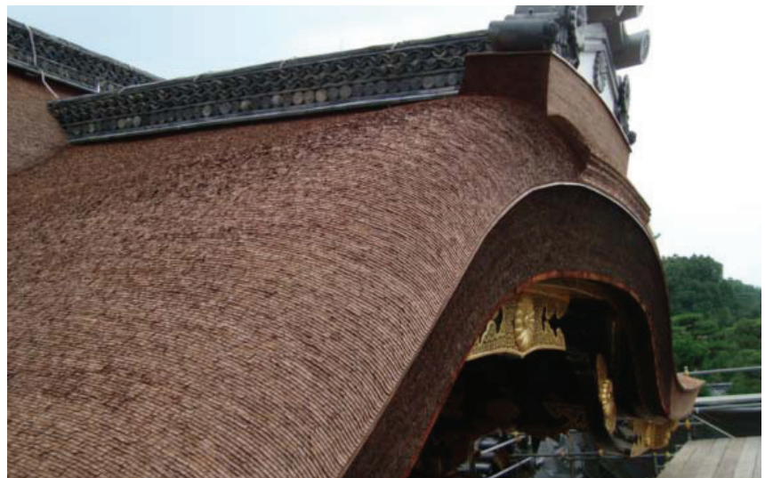
Kyoto. The restoration site of the Imperial gateway in Nijo Castle. July 30, 2013. Detail of the kara-hafu after the restoration (2013 © Olimpia Niglio).
