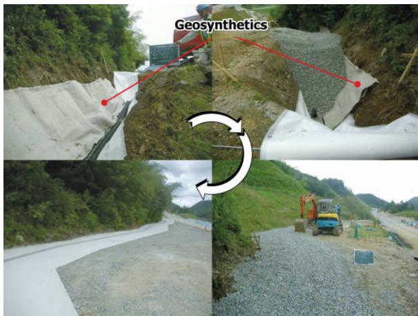
Fig. 22 Implementation of geosynthetic drain.
