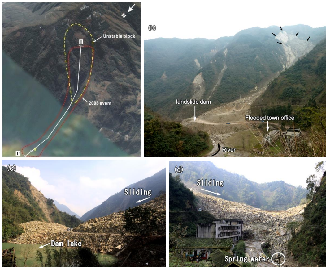
532 Fig. 2 Landslide dam in Tianchi area. (a) aerial photo of landslide area before the quake; (b) View of the 533 landslide from the upper stream of the river after all construction has been finished (Taken on March 19, 534 2011); (c) Landslide dam and lake (Courtesy of F. Cai, taken on November 7, 2008 by F. Cai) viewing from 535 upstream; (d):Landslide dam viewing from downstream (Courtesy of F. Cai, taken on November 7, 2008)
