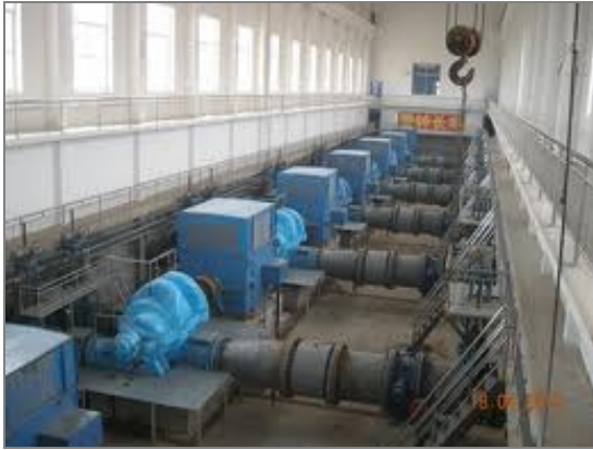
Fig 2.3 Pump station building (fucuanind)
