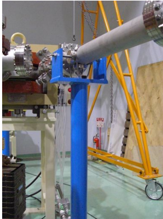
Figure 3.5: Picture of one of the support with alignment system for the collimators.
