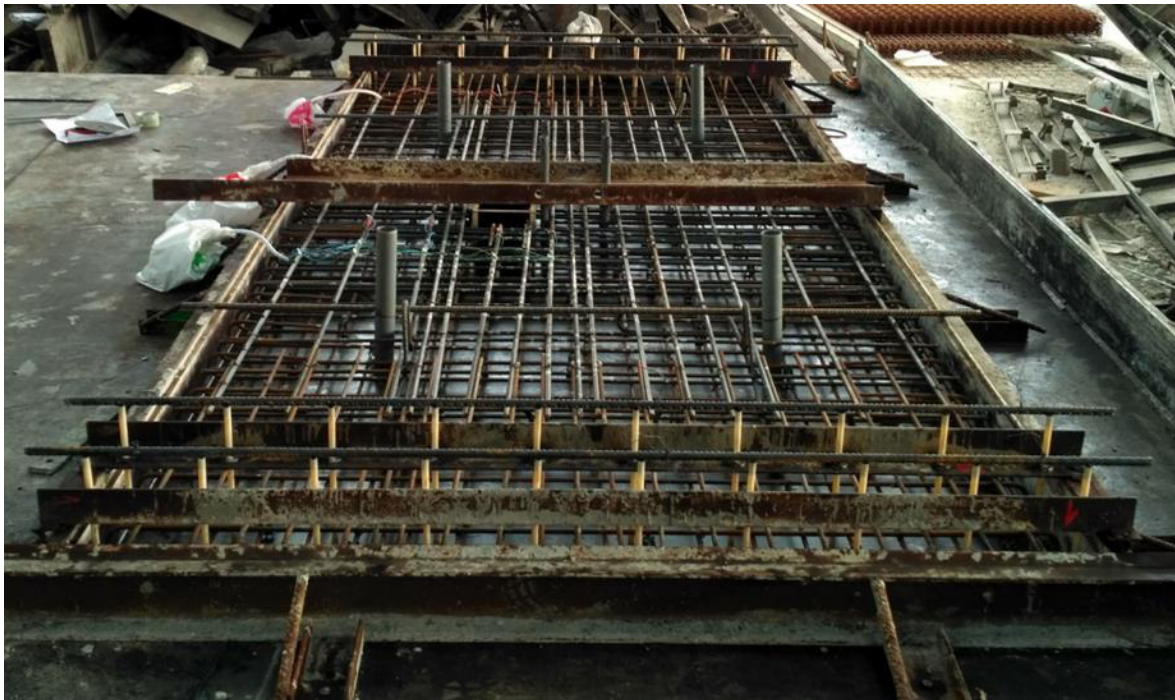
Figure 3.24 – Moulds used for the casting.
