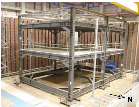
Fig. 11 General view of building specimen
