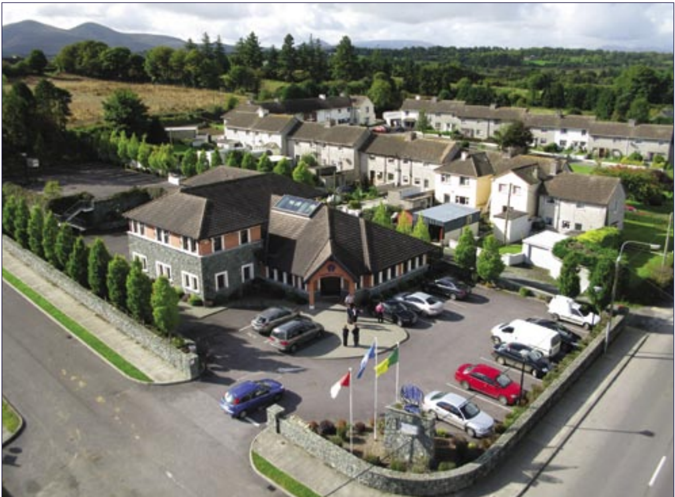
• Fig. 5 An aerial view of Rathmore Credit Union. The credit union flag is flanked by the county flags of Cork and Kerry, reinforcing the cross-county nature of the common bond. (Photo: Air Take, Meelin, Newmarket, Co. Cork).
