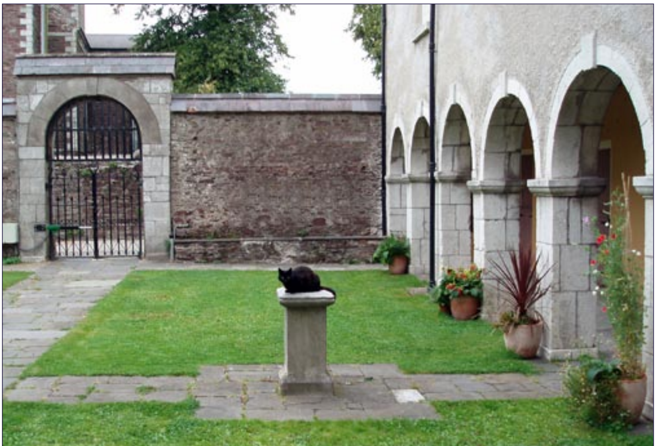
• Fig. 2 Pictured is the courtyard of Skiddy's Almshouse (with visitor), an example of a listed building restored and converted to co-operative housing (Courtesy: Cork Community Housing Co-op).
