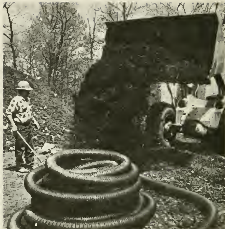
Fig. 3. A 20' x 60' bed of wood chips is laid down for good distribution of air.
