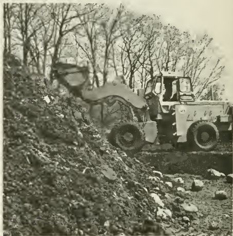
Fig. 5. The chip/sludge mixture is piled on the bed and is covered with approximately one foot of composted material for insulation.
