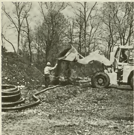
Fig. 4. Four inch perforated pipe is placed on the bed and covered with four inches of wood chips.
