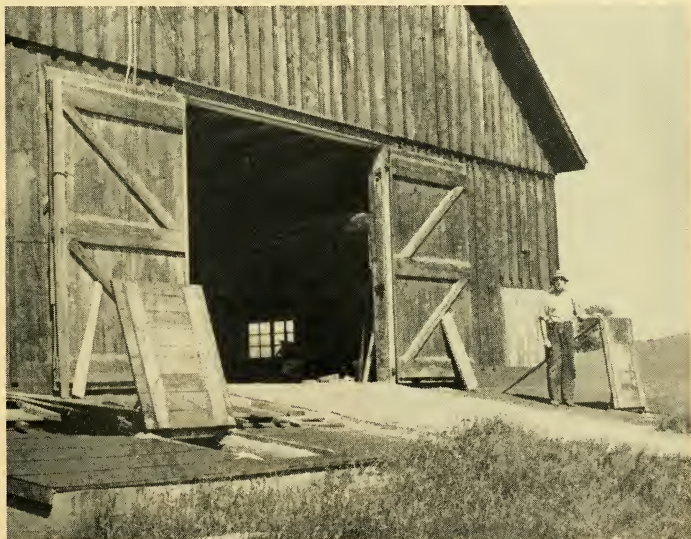
Fig. 41. This shows the trap doors leading to the sawdust storage. They are filled directly from the truck.
