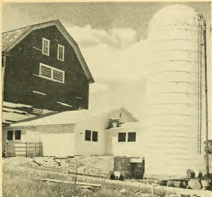
Fig. 57. In remodelling the barn, the stable was extended well beyond the old barn and adequate space was provided for a feed work center. The old barn has adequate hay capacity for the larger herd.
