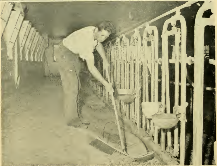
Fig. 35. This curved manger took 4.5 man minutes to sweep with an ordinary broom (above). With the curved broom (below), the time required was 2.45 man minutes.
