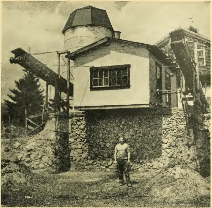
Fig. 38. This homemade barn cleaner dumps the manure on a concrete manure pit floor some distance from the barn. Under favorable conditions the operator can clean his stable in 11 minutes. He can load directly into the spreader but prefers to let it pile up and use tractor loader and spreaders in the spring and late fall.
