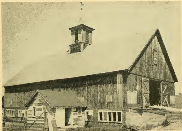
Fig. 5. A conveniently located milk house, constructed as an addition to the barn.
