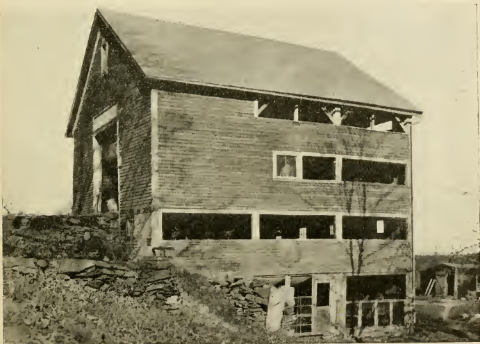
On many farms old dairy barns have been remodeled into poultry houses with three to four decks
