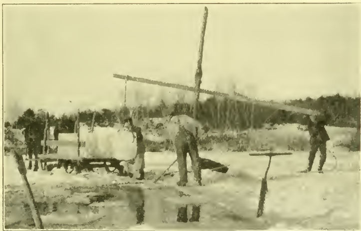
This is a chore now eliminated where electric dairy cold storage has been installed.
