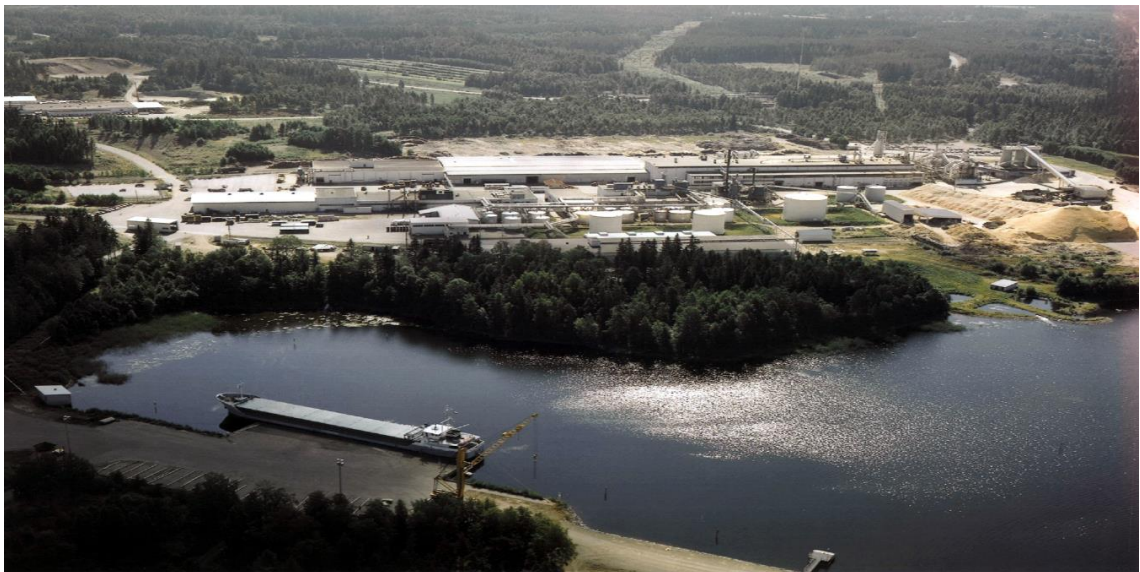
Figure 1. Puhos industrial area, Hexion Kitee site is in the middle. (Hexion 2019a)
