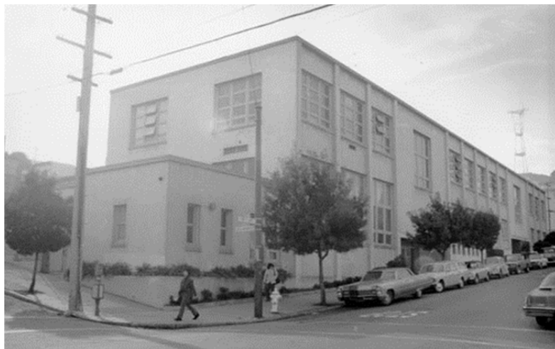
Figure 107. Douglass School, 4235 19 th Street, built 1953, photo ca. 1975. (AAD-3645, San Francisco History Center, San Francisco Public Library)
