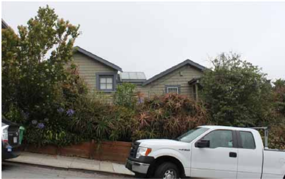
Earthquake shacks at 300 Cumberland, looking north from Cumberland
