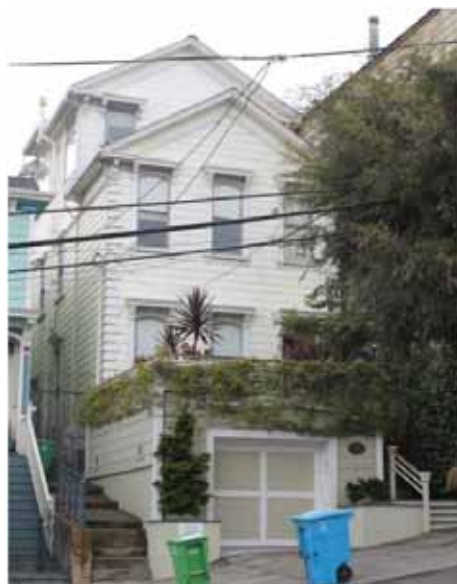
Figure 117. The earliest documented dwelling in the study area at 591-593 Noe, built 1864
