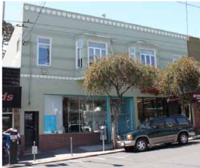
Commercial space at 4125-4131 18 th Street (built 1906, restyled after 1930)
