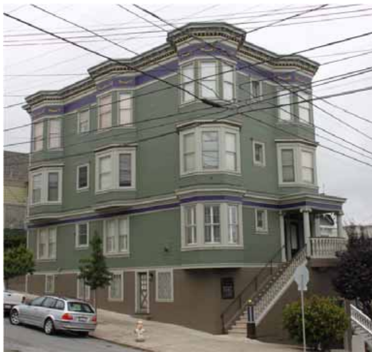
Three-flat at 294-298 Collingwood Street (built 1903)
