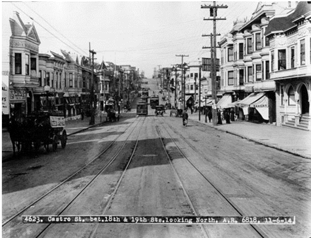
Figure 76. Castro Street between 18 th and 19 th streets, looking north, 1914. (AAB-3252, San Francisco History Center, San Francisco Public Library)
