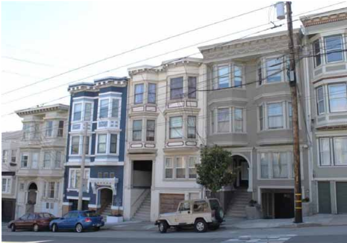
Row of three-flats at 613-615 through 627-631 Castro Street (built 1910-1913)
