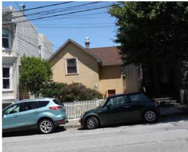
Figure 13. Dwelling associated with former Pacific Dairy, 225-227 Eureka St., ca. 1900
