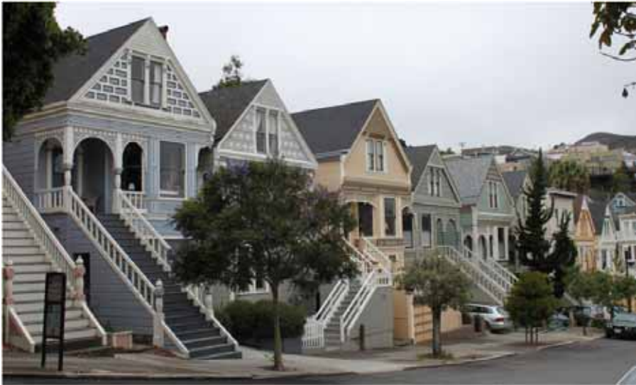
Single-family dwellings at 563 to 577 Liberty Street (built 1897)
