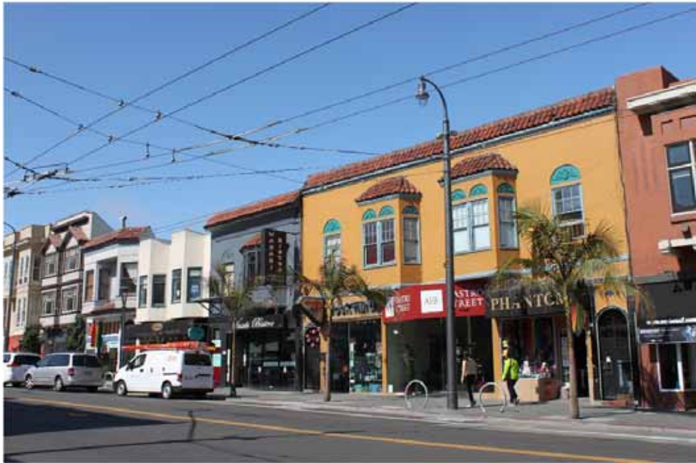
Commercial buildings at 514-526 Castro Street, built 1906-1907 with later Mediterranean Revival restyling
