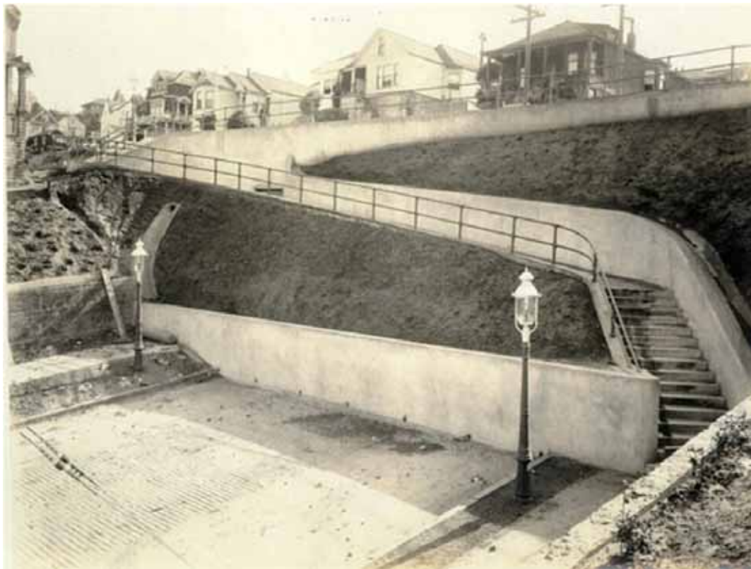
Figure 94. Cumberland Street stairs and ramp at Sanchez Street, looking west, 1916. (AAB-3354, San Francisco History Center, San Francisco Public Library)
