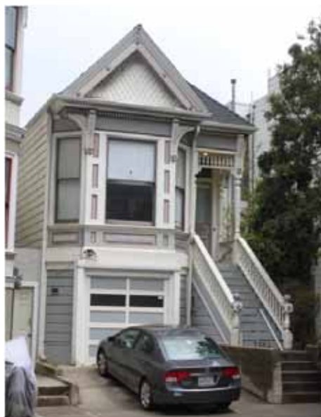
Single-family dwelling at 3964 19 th Street
