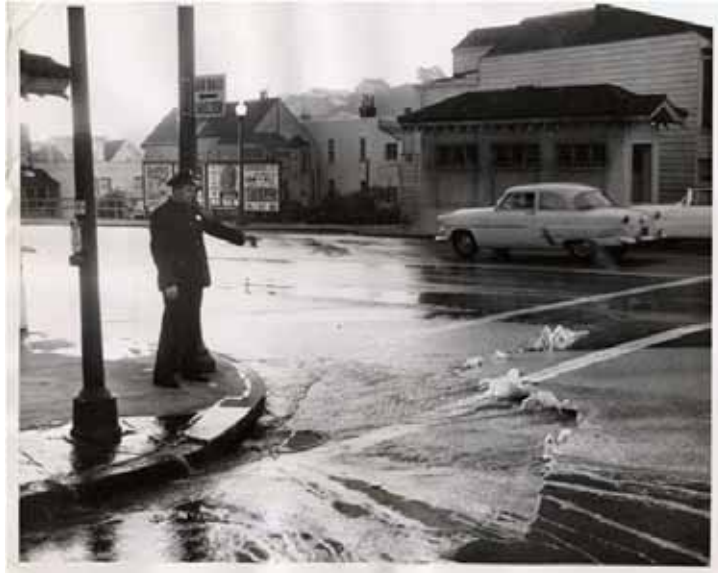
Figure 83. Eureka Street at Market Street with San Francisco Muni station head house in the background, 1956. (AAK-1044, San Francisco History Center, San Francisco Public Library)
