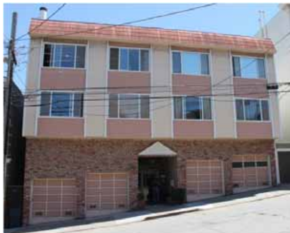
Contractor Modern apartment building, 8 units, 183 Eureka St., built 1969
