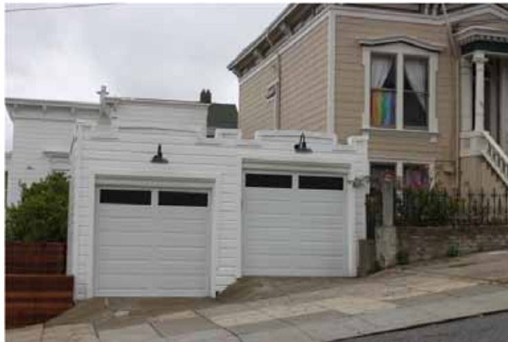
Garages associated with 183-185 Hancock Street; left garage dates to ca. 1915; right garage is after 1950, likely constructed in tandem with division of the property into two units. (Sanborn 1900, 1914, 1950)
