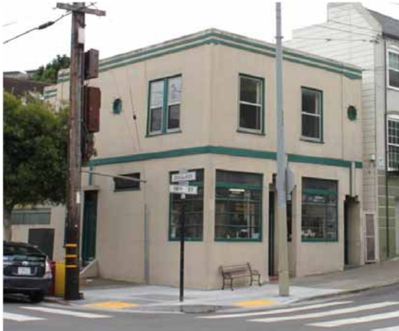
Commercial space and flat at 4103-4105 18 th Street (built 1906, remodeled ca. 1930)
