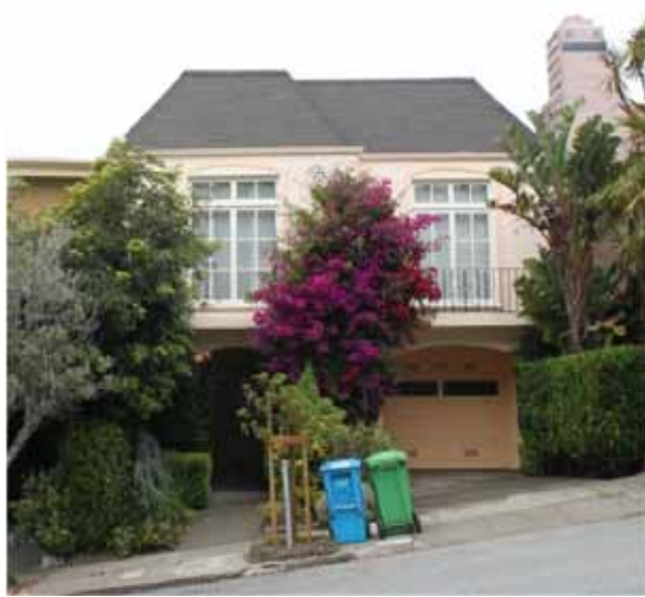
Single-family dwelling at 348 Cumberland Street (built 1939)
