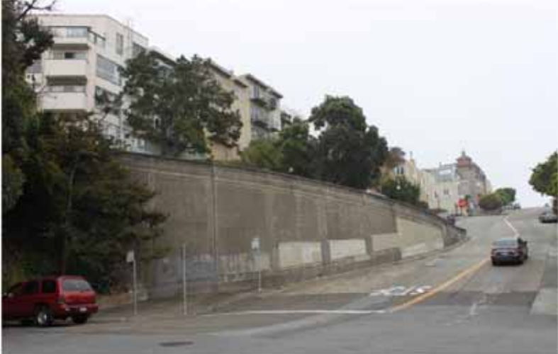
Figure 95. Retaining wall along 20 th St. at Noe St., looking south
