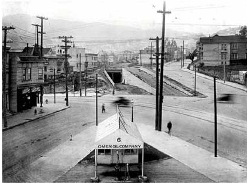
Figure 81. Twin Peaks Tunnel nearing completion, ca. 1917 (Private Collection, San Francisco, CA; published online at Found SF, http://FoundSF.org/index.php?title=New_Tunnel_1919 )
