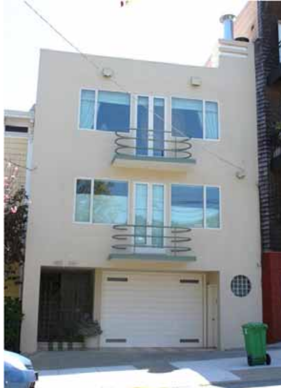
Two-flat at 189-191 Collingwood Street (built 1940)
