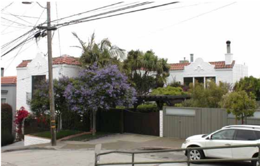
Two-family dwelling at 377-379 Collingwood Street (built 1931)
