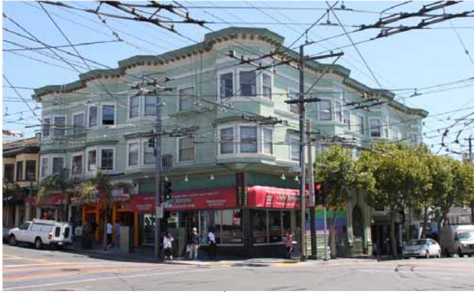
4092-4096 18 th Street (built 1905)
