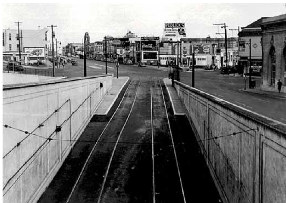
Figure 79. Market Street commercial district from the Twin Peaks Tunnel, ca. 1930. (Private Collection, San Francisco, CA, published online at Found SF, http://FoundSF.org/index.php?title=Twin_Peaks_Tunnel )
