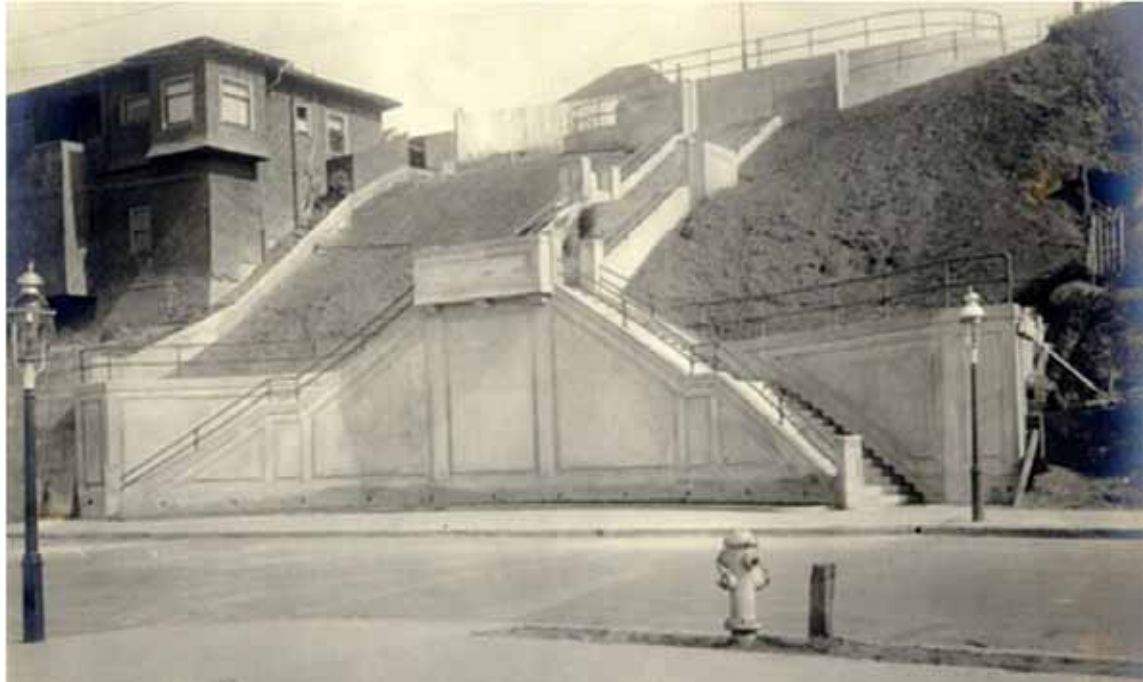
Figure 93. Sanchez Street retaining wall and staircase, looking south from 19 th Street. (AAB-3355, San Francisco History Center, San Francisco Public Library)
