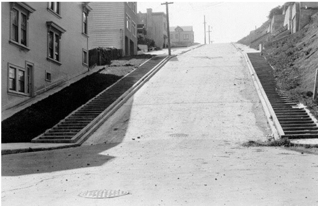
Figure 89. Collingwood Street sidewalk steps at 20 th Street, looking south, 1926. (AAB-3384, San Francisco History Center, San Francisco Public Library)
