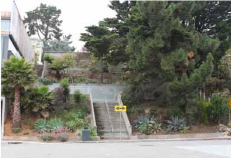
Figure 96. 20 th St. Stairs at Sanchez St., looking west
