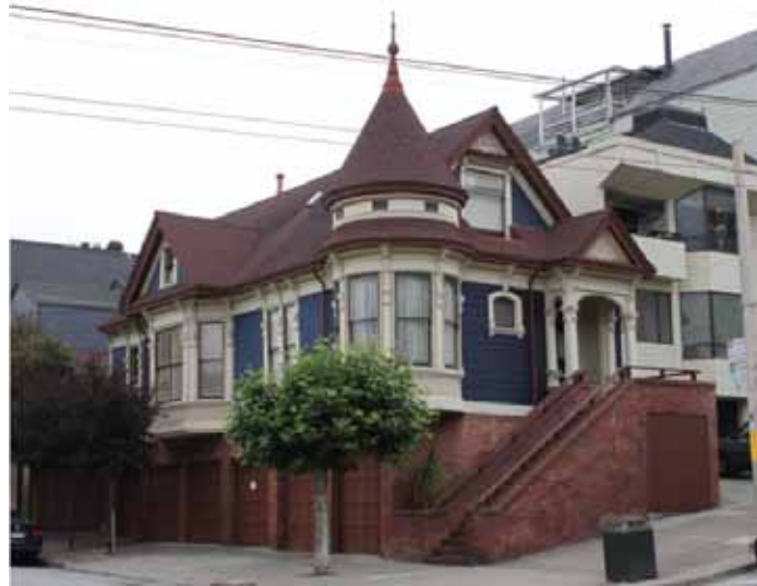
Figure 43. Fernando Nelson House, 701 Castro Street (built 1897)
