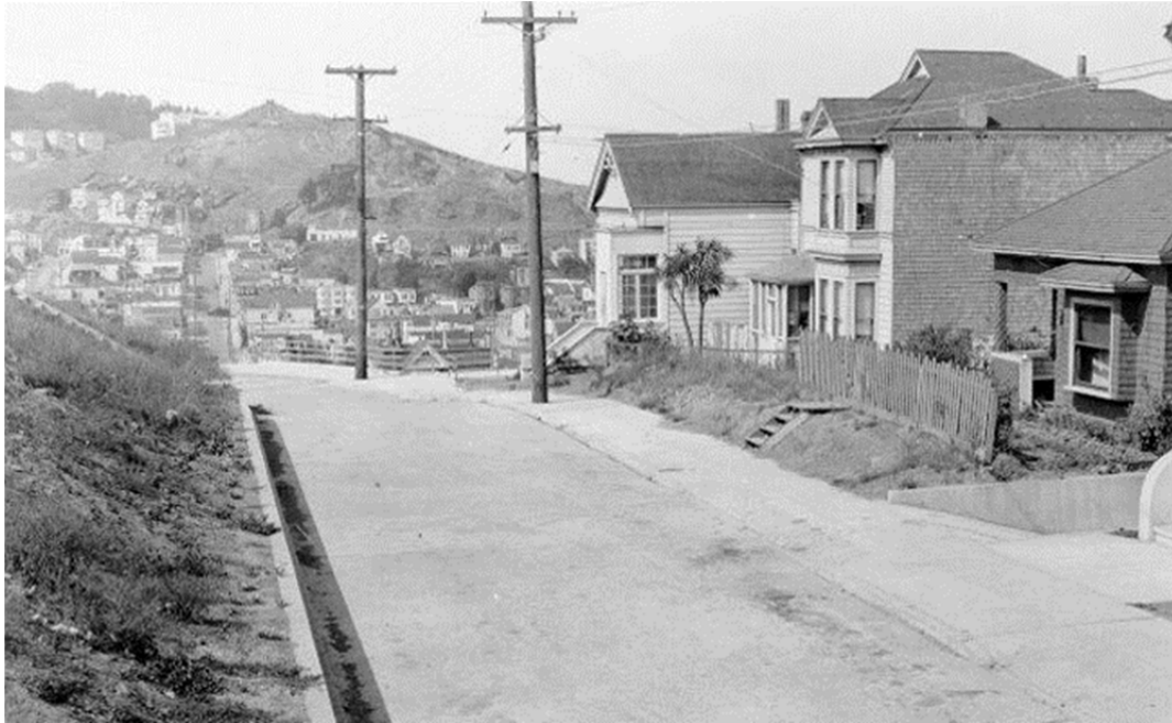
Figure 91. Douglass Street looking north toward 20 th Street retaining wall and pipe railing, 1927. (AAB-3386, San Francisco History Center, San Francisco Public Library)
