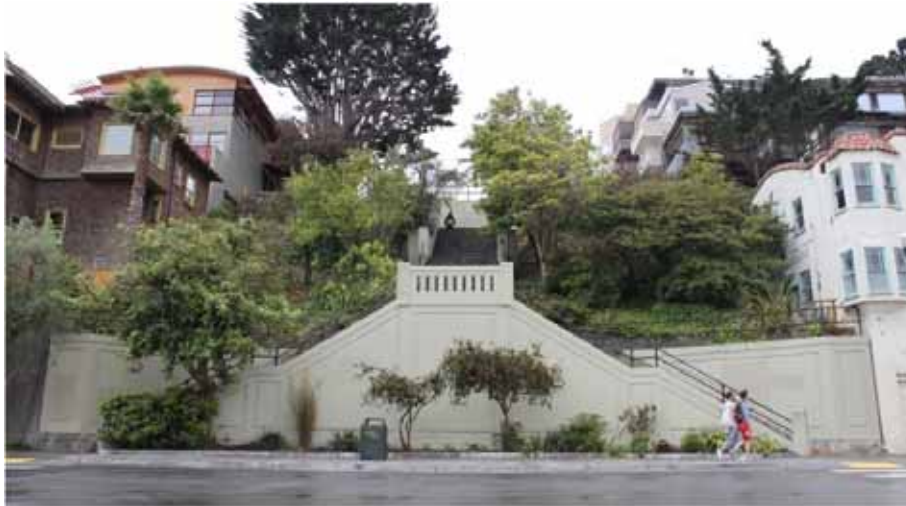
Figure 99. Retaining walls and pedestrian stairs at Sanchez and 19 th streets
