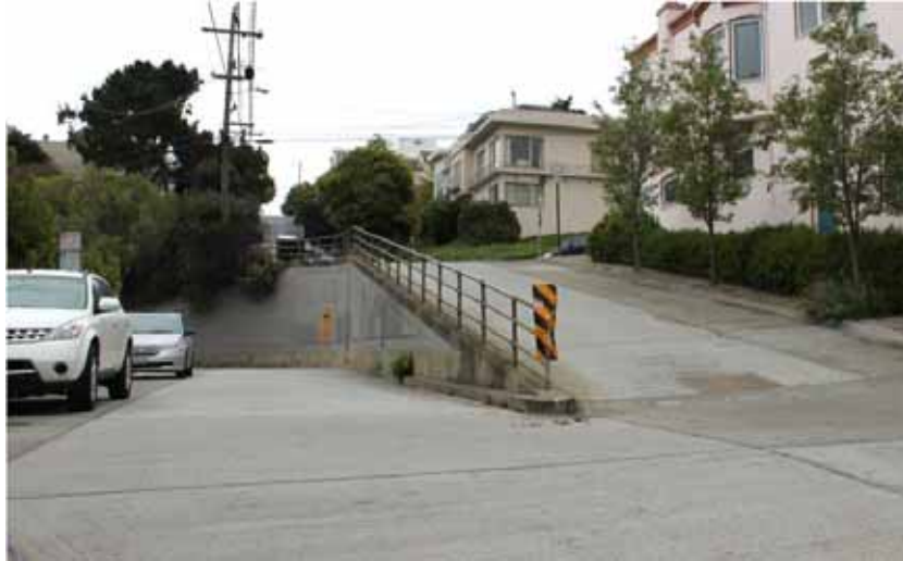
Figure 98. Collingwood Street retaining wall and switchback onto 21 st Street
