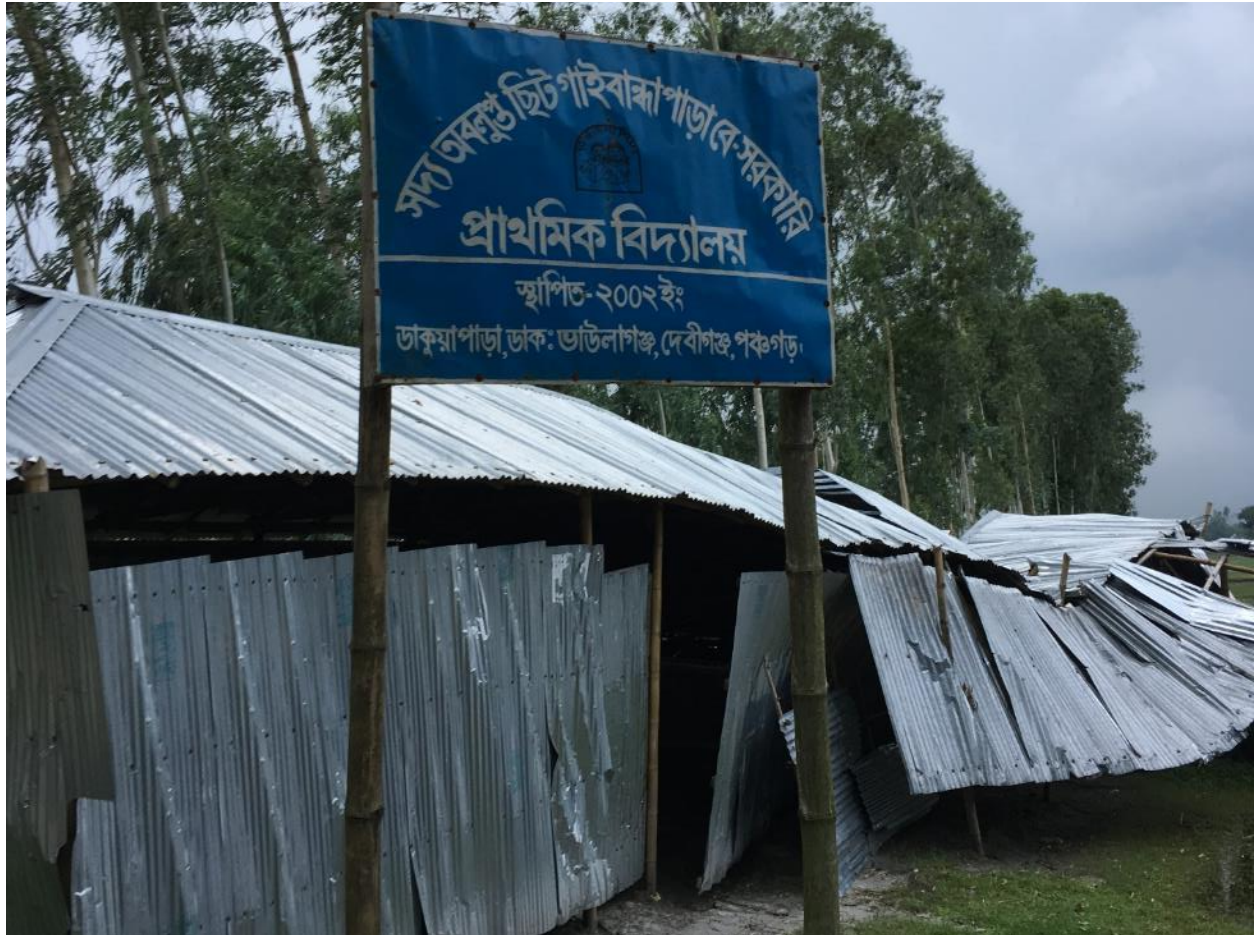
Figure 16: The abandoned school in the Gaibandha Para
