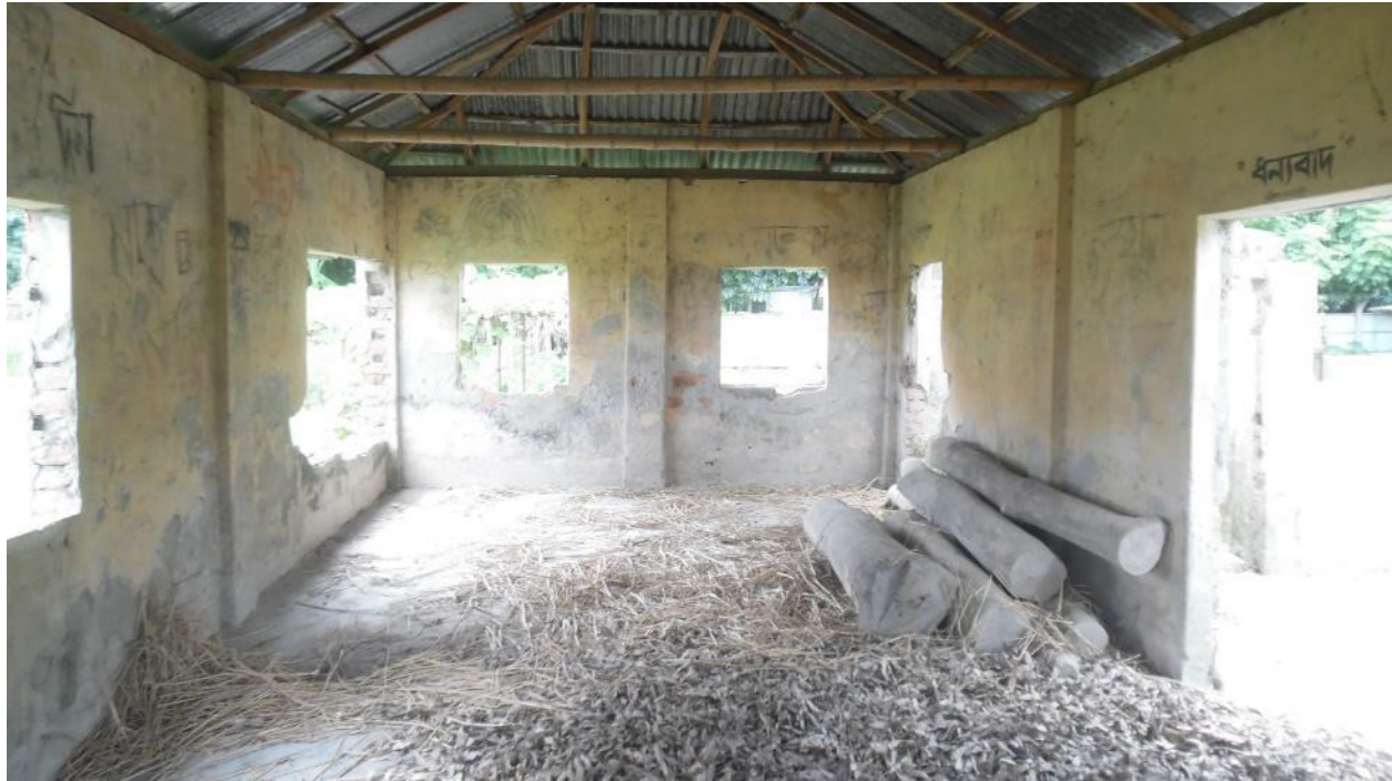
Figure 7: The abandoned office and courtroom of the Dasiar Chhara chhit council
