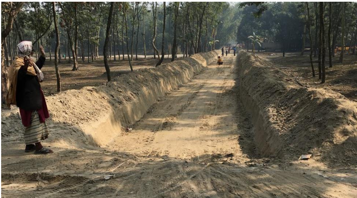
Figure 4: Exploring the road construction on the first day in Balapara Khagrabari
