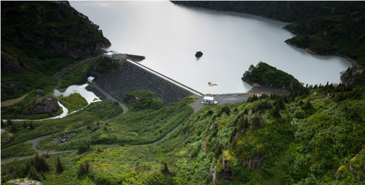
Bradley Lake Dam
