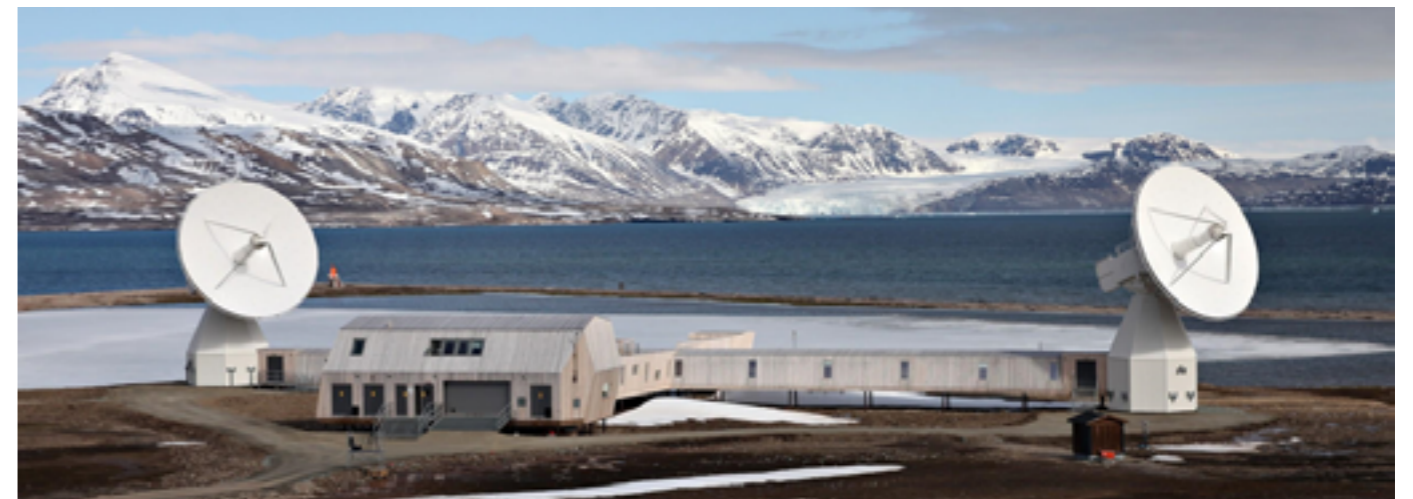
Figure 3.6.2 The Earth observatory at Ny-Ålesund which is a core geodetic site, i.e. a number of different geodetic instruments are collocated. The site is part of a global network that is of fundamental importance for determining accurate measurements of sea level from satellite altimetry. The twin VLBI telescope is pictured. Photo: Bjørn-Owe Holmberg
