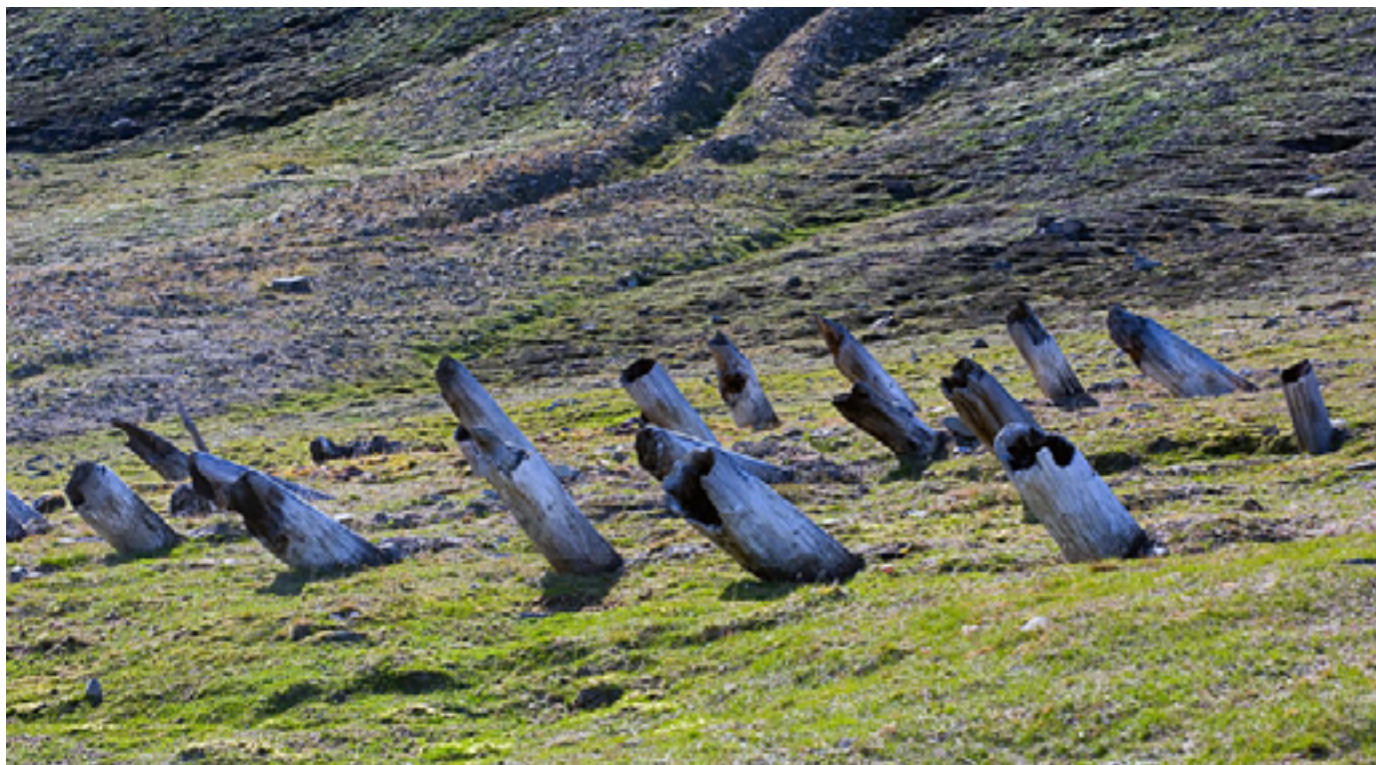
Figure 7.2.1 Solifluction is evident in Longyearbyen where posts formerly used as foundations of houses have tilted downslope (Photo J. Alean, Swissheduc.ch)
