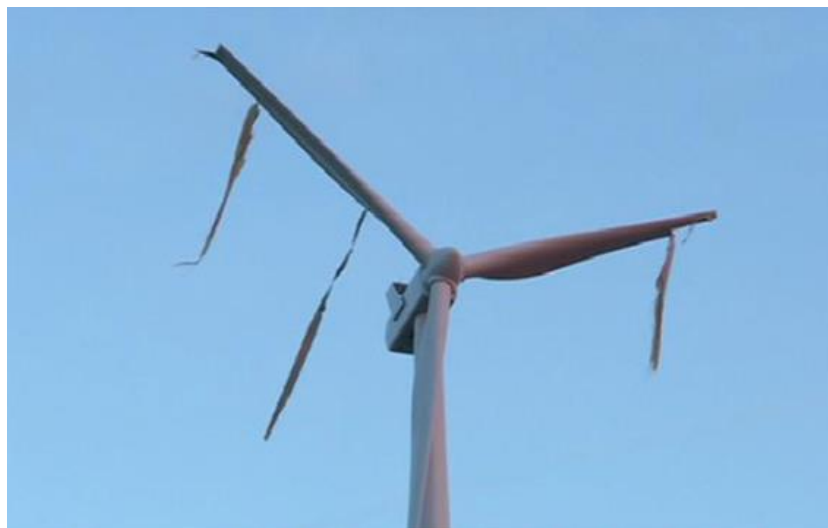
Figure 2-17 Structural failure due to faulty manufacturing (Dongsheng, et al., 2015)
