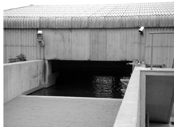
Fig.3. Monitoring cameras which were fixed on the upper side tank wall connected to the nesting bed
