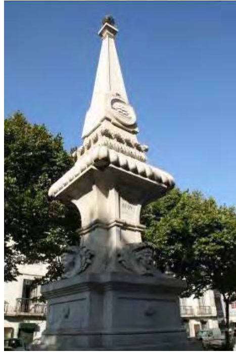
Chafariz de S. Paulo one of the still existing stone fountains
