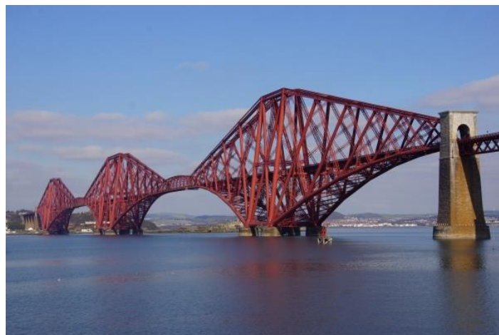
Figura 23 - Ponte Firth of Forth (Nicolas Janberg, 2016).
