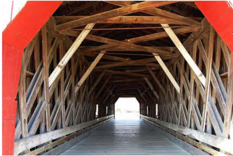
Figura 13 - Lattice Truss, Minnesota (MARINHO, 2012).
