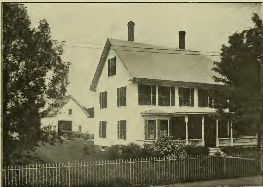
Residence of Stephen A. Frost.
