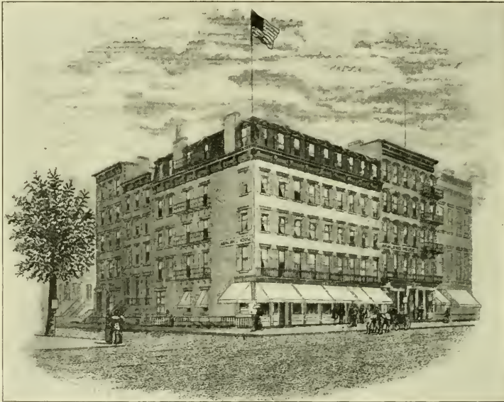
Ashland House, New York City
