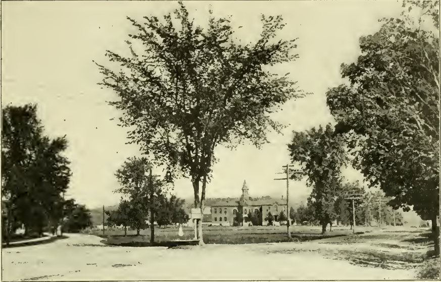
Cheshire County Jail
