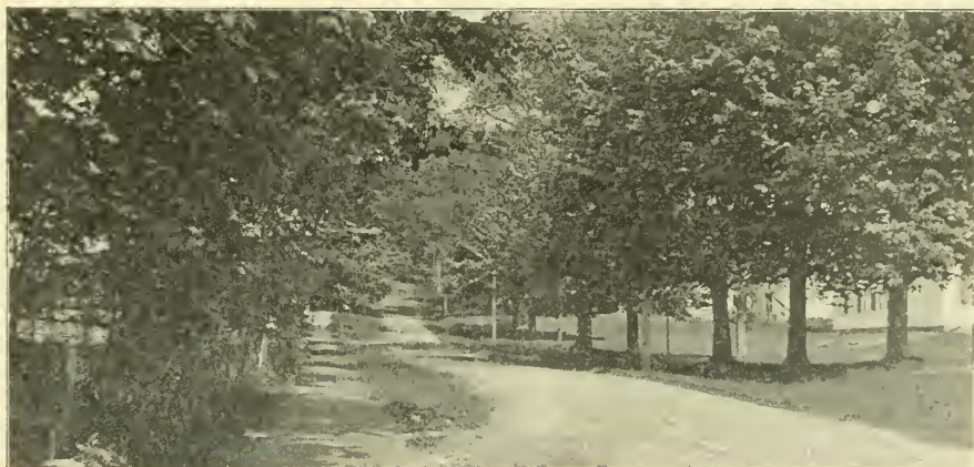
Street leading to Seminary Hill, Gilmanton Corner
