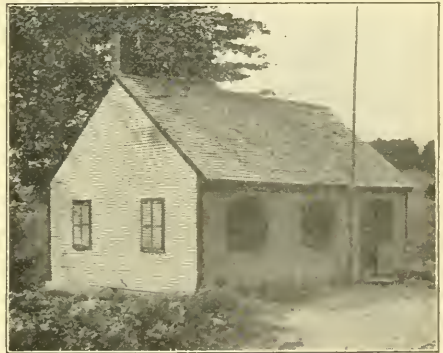
School House—Dist. No. 7
